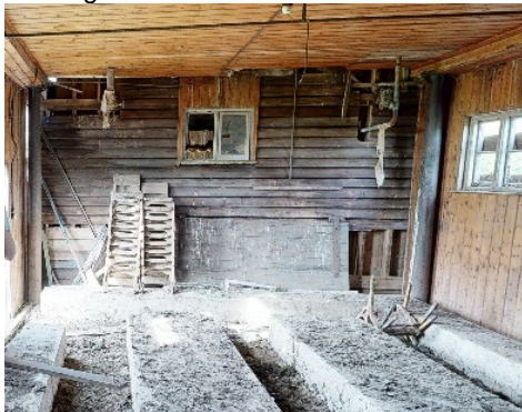
Internal Wall (Original South Elevation)
