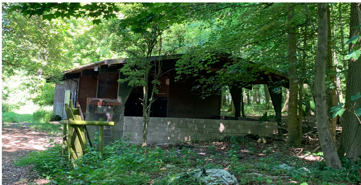
Existing Summerhouse Plantation building
