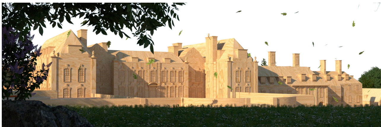
Main Building, south elevation
