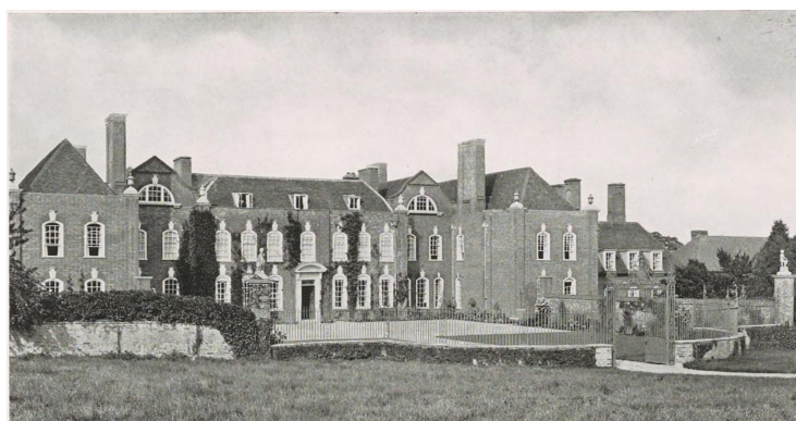
FIG. 373.—THE ENTRANCE FRONT.
