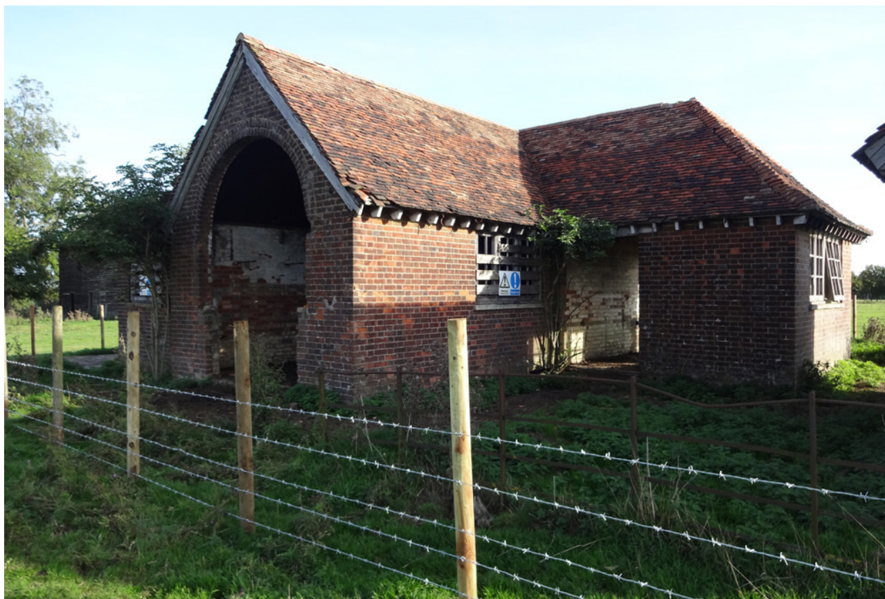
(above) Pump House, 2024
