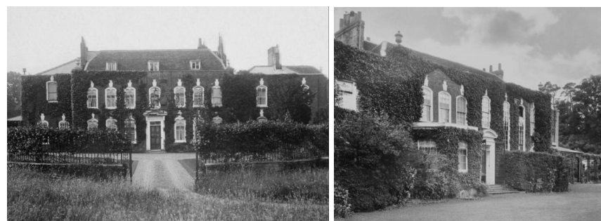
Photos of front and rear elevations of central block pre EC20 Lutyens works.
