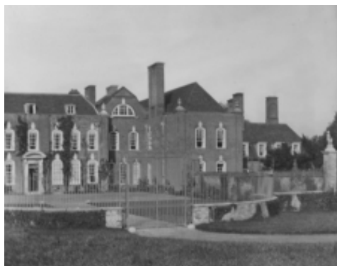
Photo of front south elevation showing EC20 Lutyens additional East Wing.
