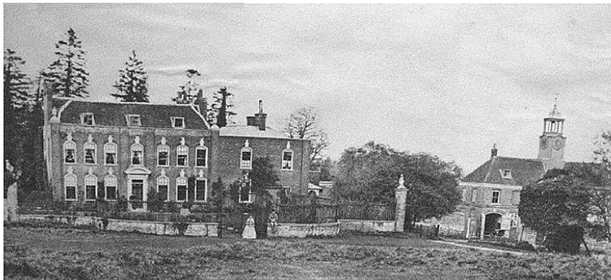
Mid 19 photograph showing the Stable Block with the large central clock tower that was later destroyed in a fire, in 1888. Notice the lack of chimney stacks to the roof of the Stable Block and the large coach doors that were mirrored on the East end.
