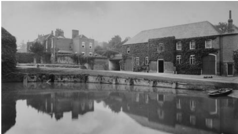
Late C19/Early C20 photograph taken of the Pond and Stable Block at Temple Dinsley prior to Lutyens' 1909 alterations.
