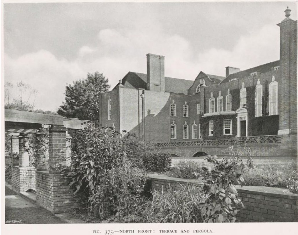
The North Terrace c.1912 showing low planting on the various terraces. The left-hand bay window on the 18 th century central block had a yew “canted bay” on the right for the sake of symmetry, This conceit predated Lutyens. L Weaver, Houses and Gardens by Sir Edwin Lutyens, 1913pp 223
