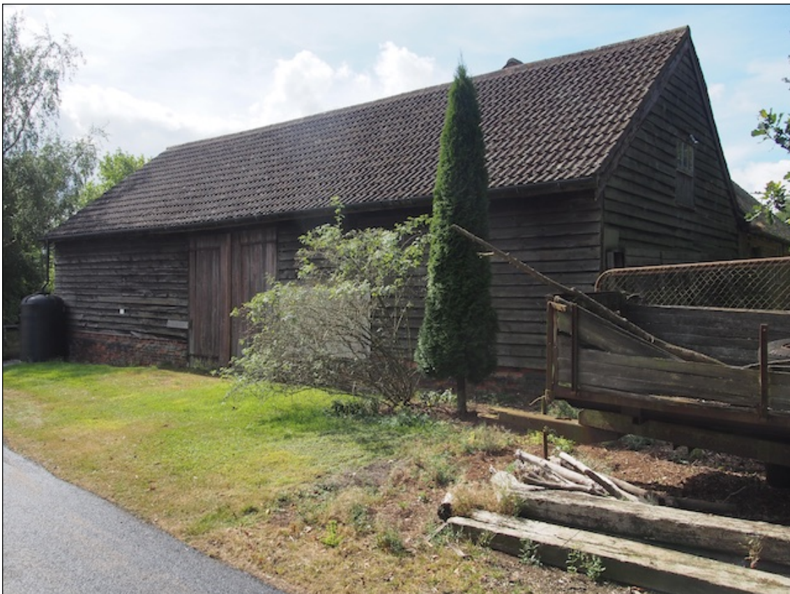
Photo 10: Front and gable elevation of the former cart-shed fronting the road
