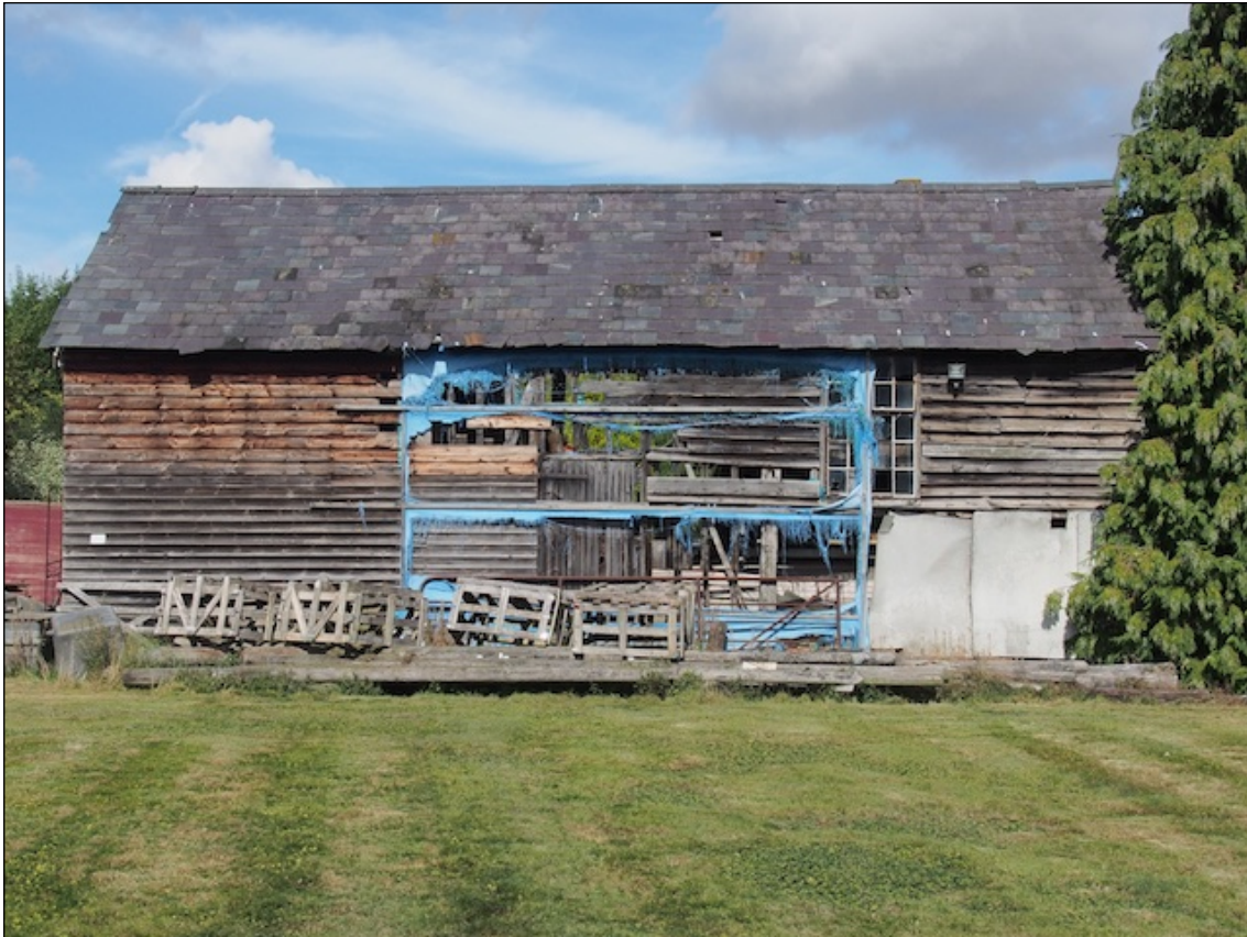
Photo 5: Rear elevation of the former threshing barn with a possible earlier opening outlined by the blue plastic sheeting
