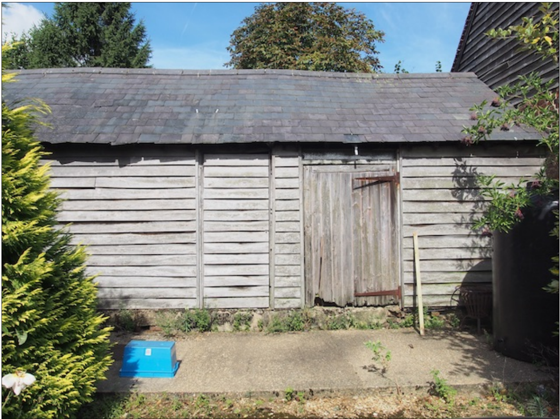
Photo 13: Front and gable elevation of single storey building
