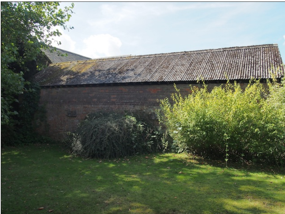
Photo 2: Rear elevation of the stables/looseboxes
