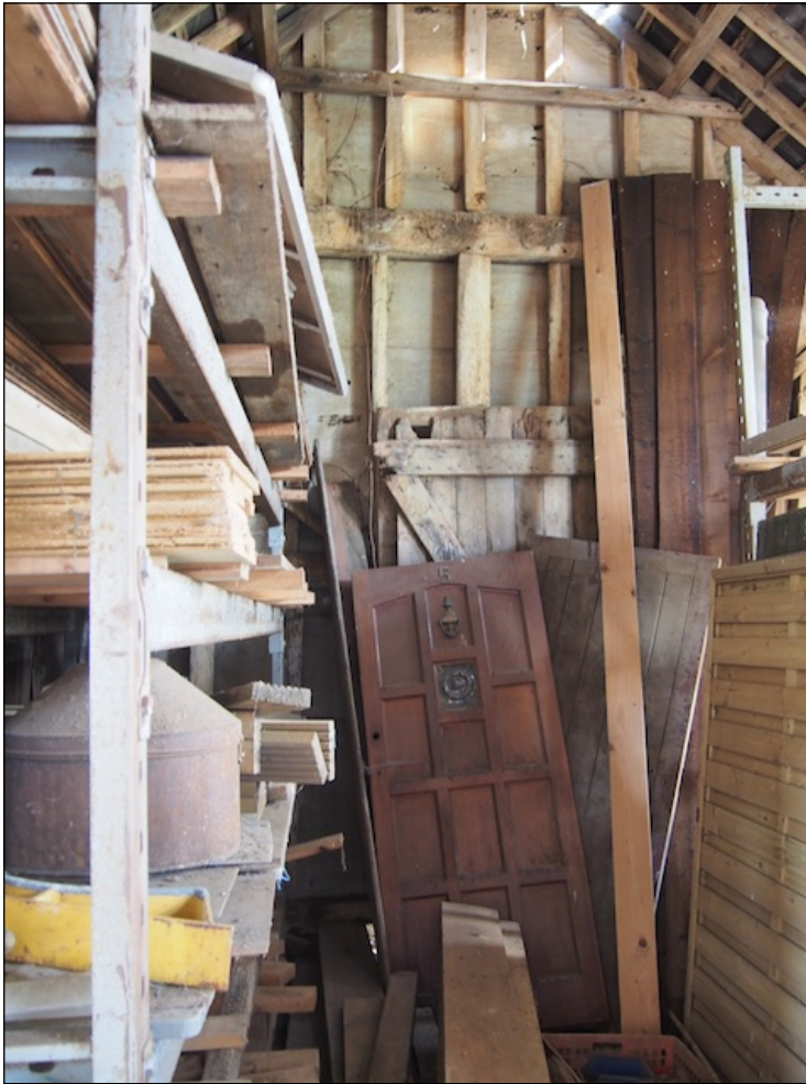
Photo 7: Internal view within the former threshing barn showing timber framing
