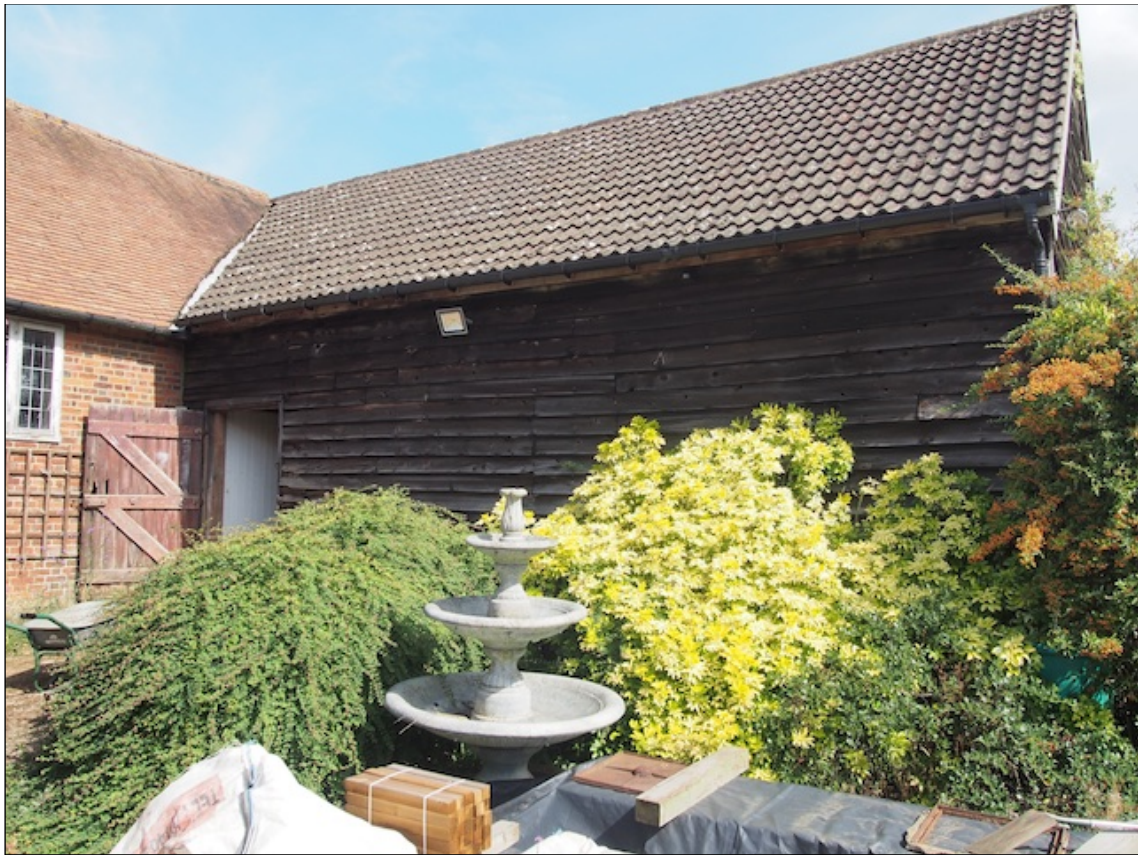
Photo 11: Internal (rear) elevation of the cart-shed
