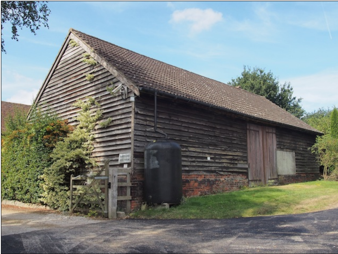
Photo 9: Front elevation of the former cart-shed fronting the road
