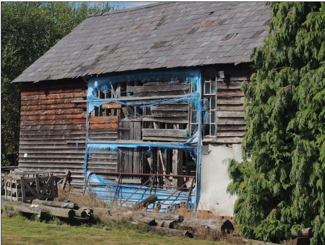
Photo 6: Detailed view of the rear elevation of the former threshing barn showing existing openings and outline of a possible earlier opening
