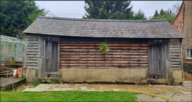
HENHOUSE FRONT ELEVATION showing existing doors retained as shutters with glazed secondary door
