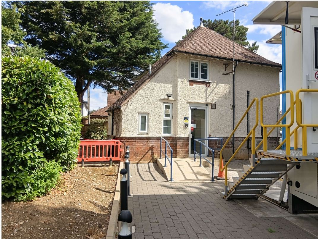
PHOTO 1 LOOKING TOWARDS LODGE ENTRANCE
