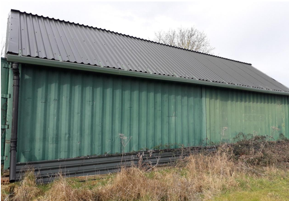
Photograph 2: Building 1, eastern aspect
