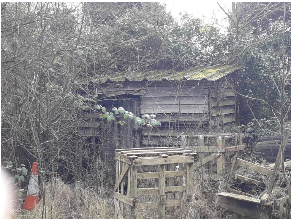
Photograph 5: Building 3, northern aspect
