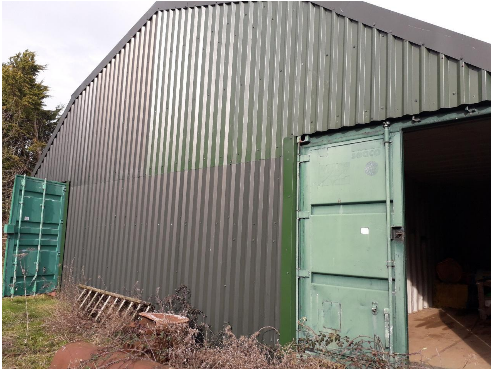
Photograph 1: Building 1, southern aspect
