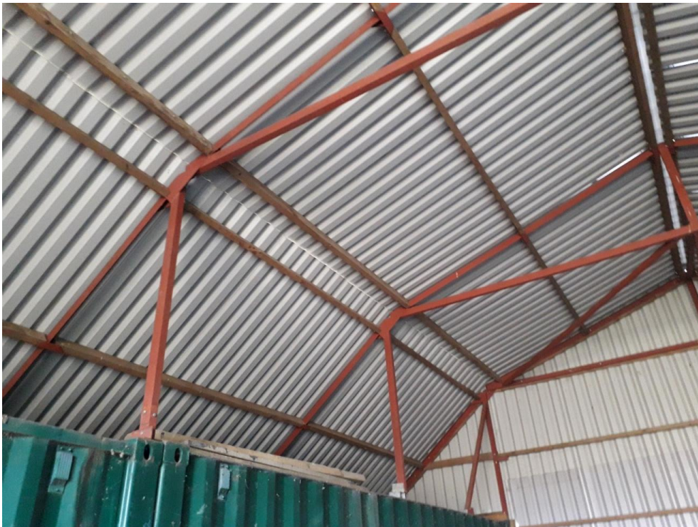
Photograph 3: Building 1, internal view
