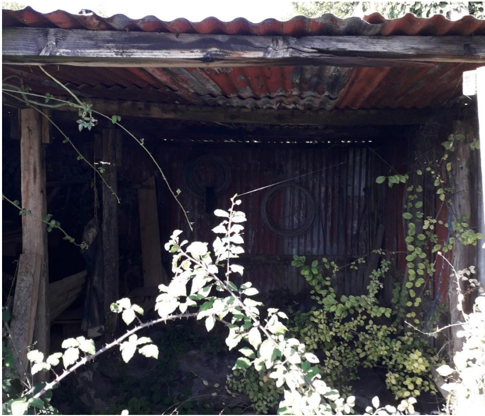
Photograph 6: Building 4, eastern aspect
