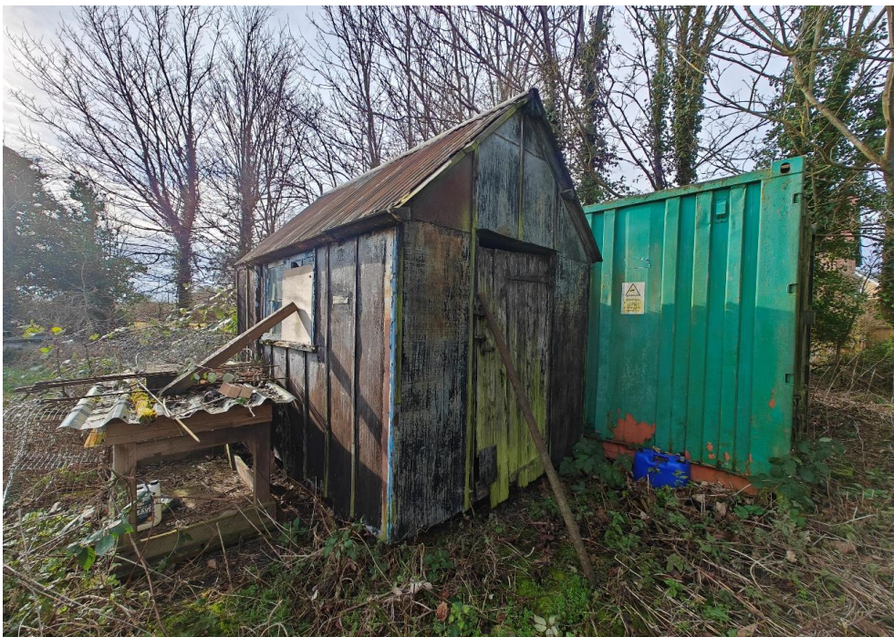
Photograph 4: Building 2, northern aspect
