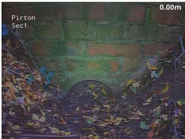
1, 00:00:00, 0.00 m Start node, outfall, reference: HW1
