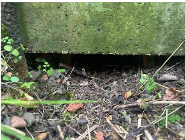
HW2 pipe soffit not visible
