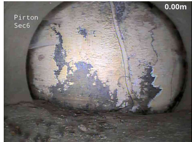
2, 00:00:16, 0.40 m Finish node, manhole, reference: B, Capped, assumed for future use
