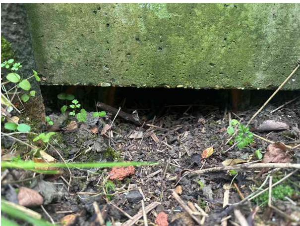
HW2 pipe soffit not visible
