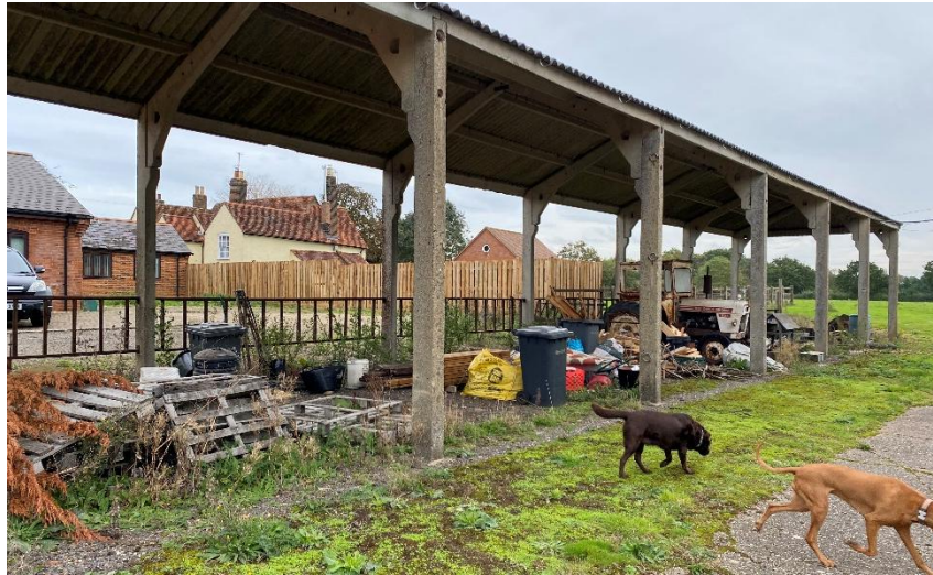
Photograph 5: View looking northwest towards Titmore Green Farmhouse; concrete framed agricultural storage barn to be re-clad in stained timber weatherboard over a brick plinth to provide ancillary storage space. Existing business units at Titmore Court (left of picture).
