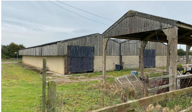
Photograph 1: View looking south showing agricultural buildings proposed for conversion to residential and business use. The buildings have planning permission to change to Class E (g)(iii) light industrial and B8 storage use. Concrete framed open barn (right of picture) to be re-clad and retained.
