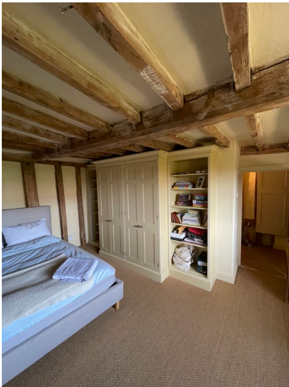
Photo 9.1 - modern cabinets to be removed.
