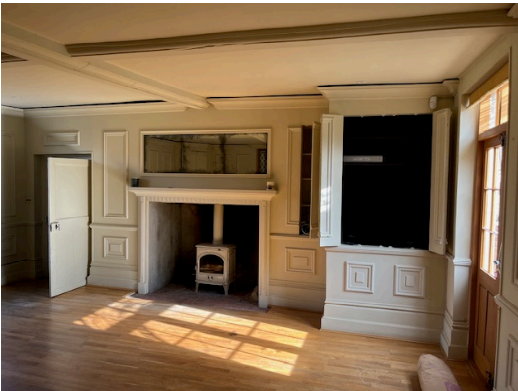
Photo 1.2 - modern wall panelling, modern cornice, modern fire surround and modern cabinet to be removed.
