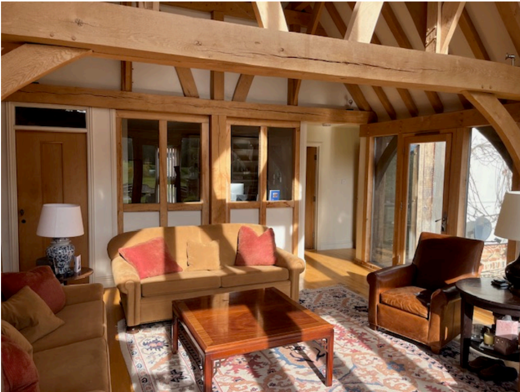
Photo 5.1 - partition and redundant non-structural oak brackets to be removed.
