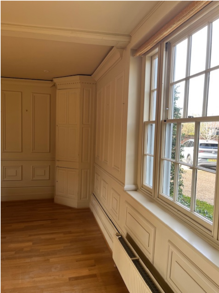
Photo 1.5 - diagonal corner cabinet to remain, modern wall panelling and cornice to be removed.
