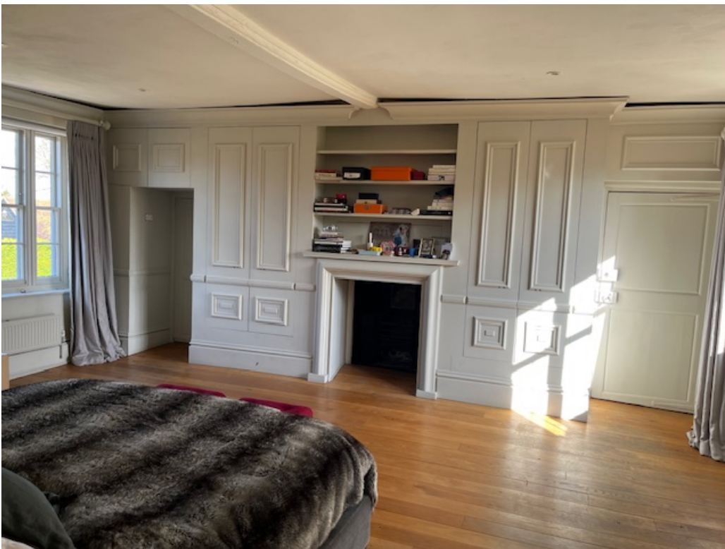
Photo 7.2 - modern cabinets and fire surround to be removed (N.B. upmost care will be taken during the removal of the fireplace surround as it is thought this could be historic fabric), floor construction to be investigated.
