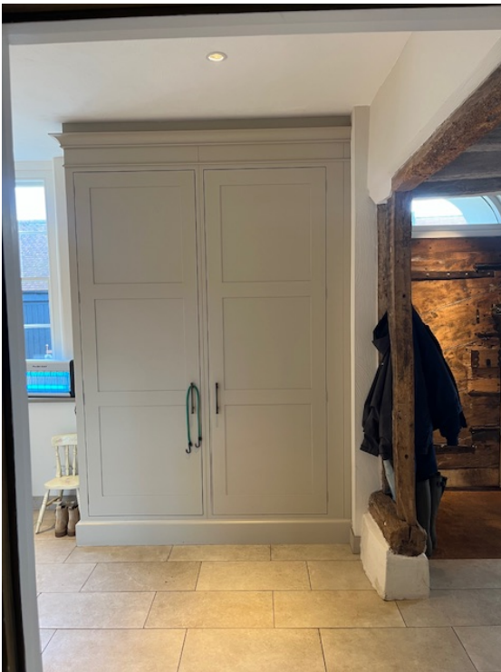
Photo 3.2 - modern cabinets and modern skirtings to be removed.
