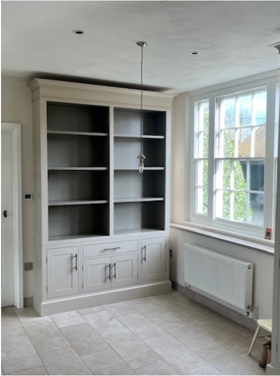
Photo 3.1 - modern cabinets and modern skirtings to be removed.
