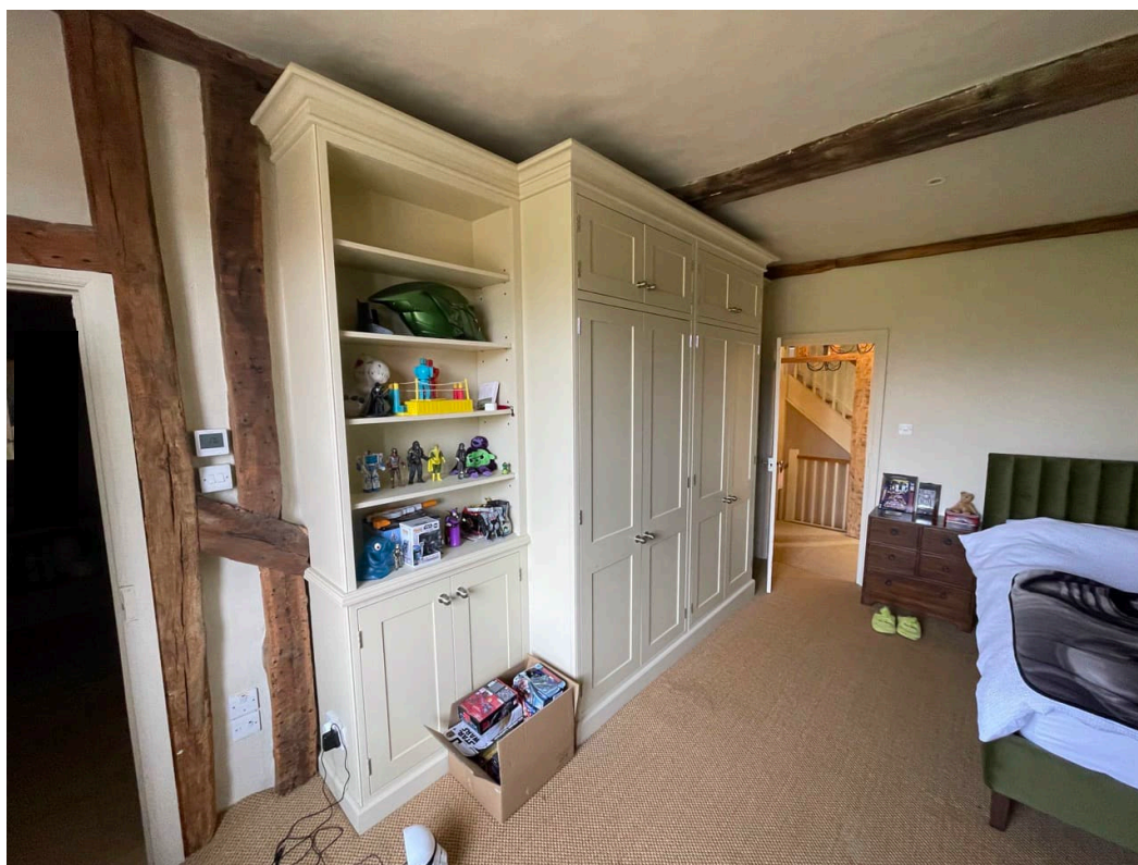
Photo 8.1 - modern cabinets to be removed.
