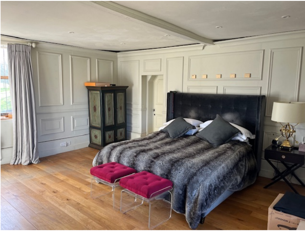
Photo 7.3 - modern wall panelling to be removed.
