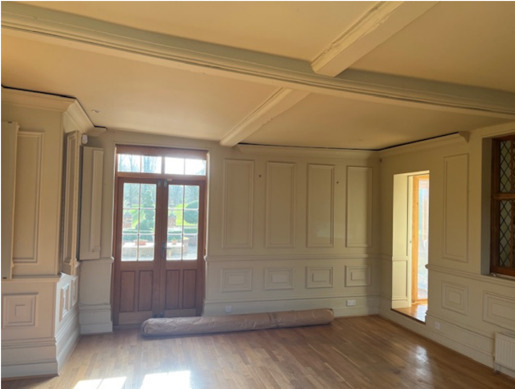
Photo 1.3 - modern wall panelling, modern cornice and modern cabinet to be removed.
