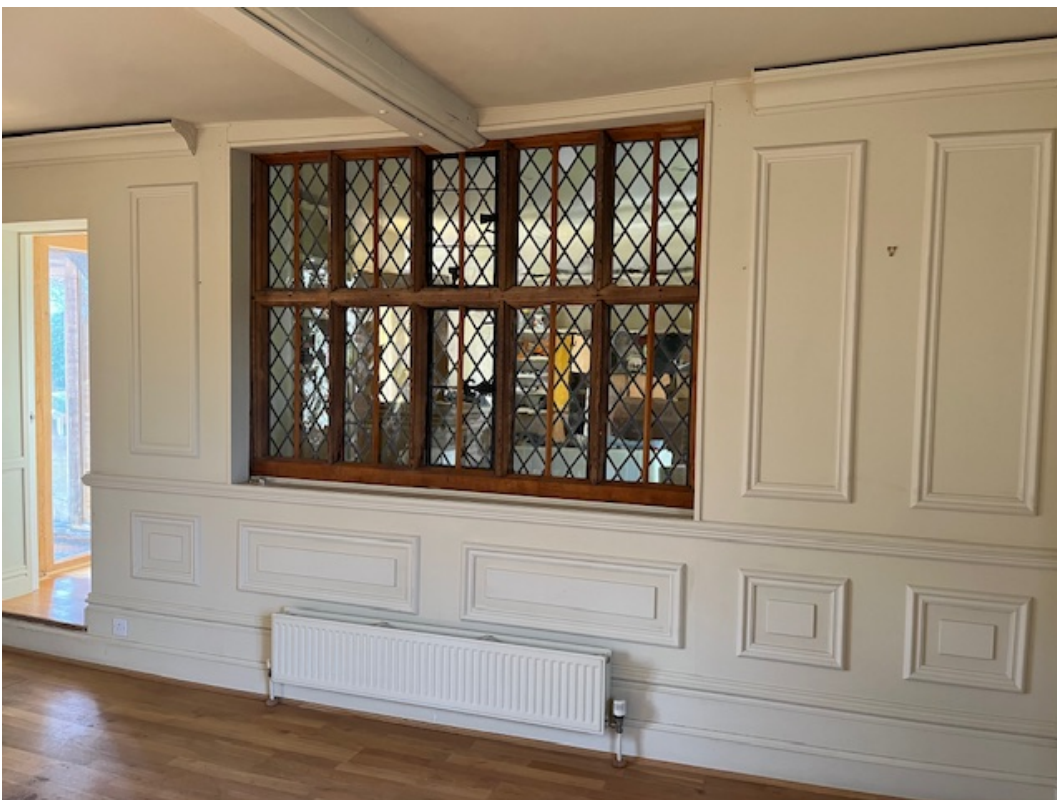
Photo 1.4 - modern wall paneling and modern cornice to be removed.
