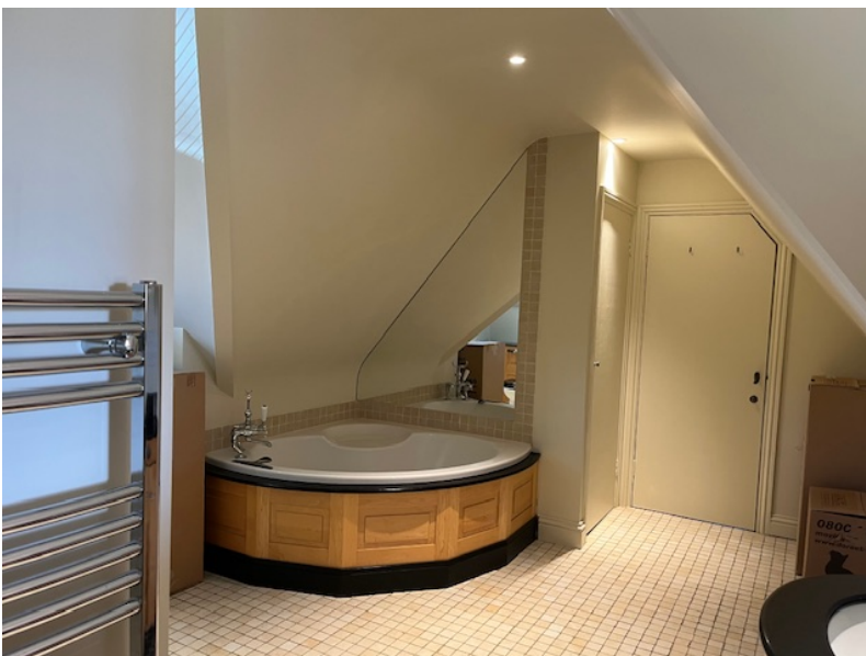
Photo 6.2 - master bathroom to be stripped out.
