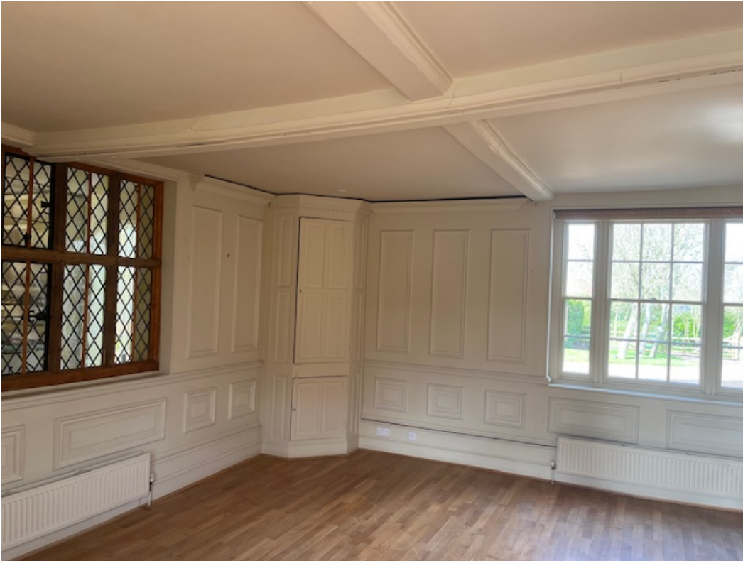
Photo 1.1 - diagonal corner cabinet to remain, modern wall panelling and modern cornice to be removed.
