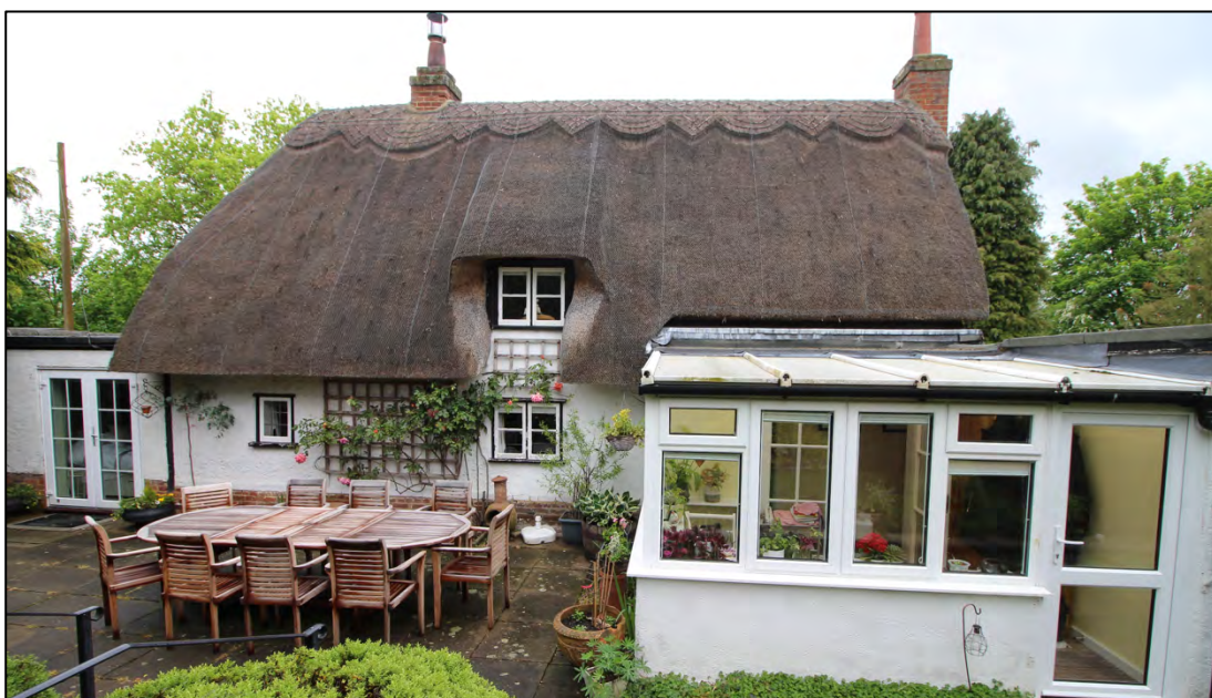
Figure 3 - Existing Photograph Rear Elevation
