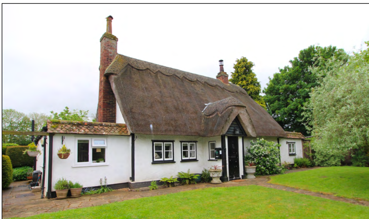
Figure 2 - Existing Cottage from Maiden Street
