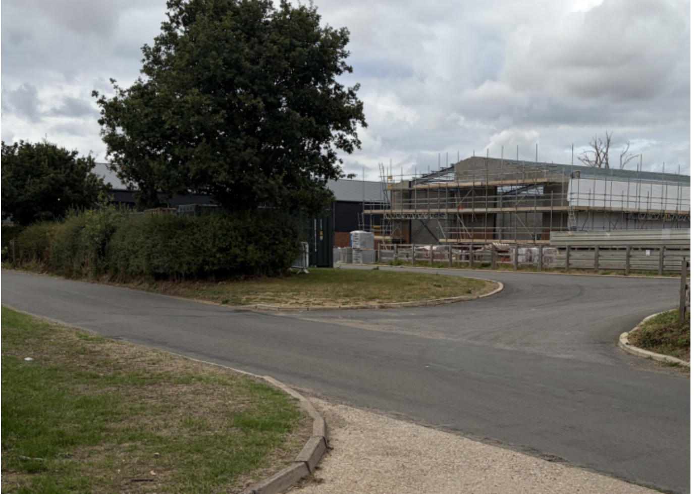
P1 - Park Lane, from the Nup End Business Centre access, looking west
