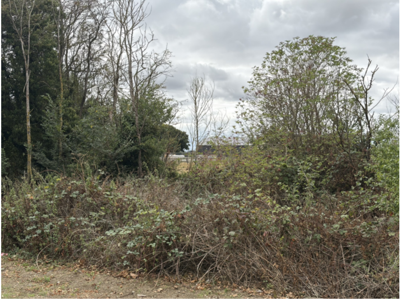
H2 - Park Lane, beside the electricity substation, looking south-west
