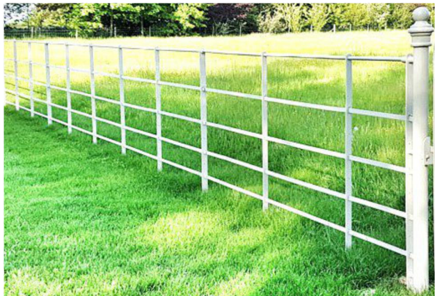
Estate fencing 900mm high (finished in Ivory colour) with traditional cast iron posts and finials
