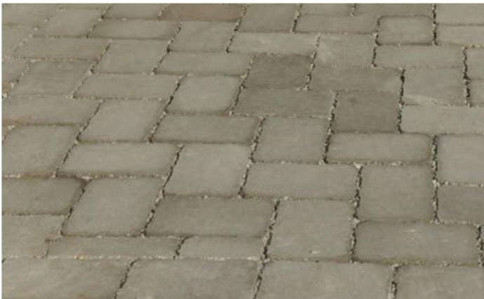
Hydropave Tobermore Tegula 240 x160 x 80mm in slate colour, laid in herringbone pattern to courtyard areas
