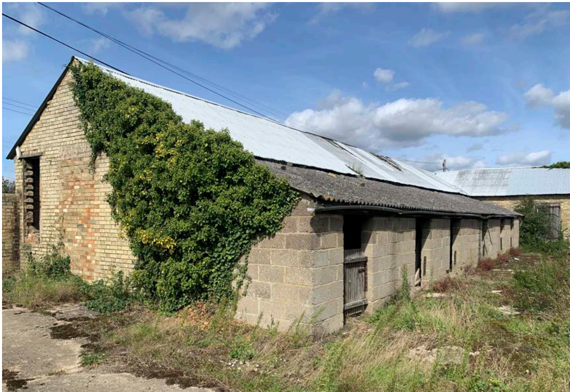
Figure 9. South and east elevations of west wing
