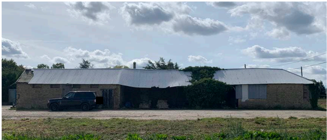
Figure 7. North elevation of north wing
