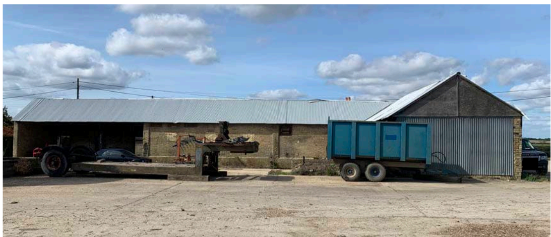
Figure 8. East elevation of east wing
