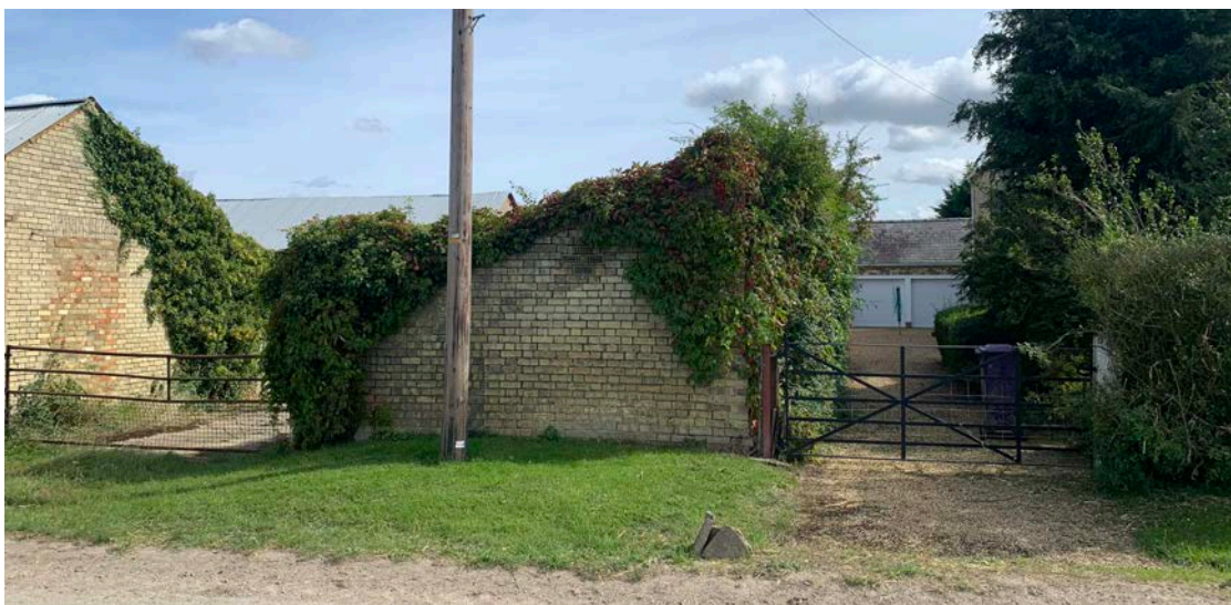
Figure 12. West elevation (Northfield Road)
