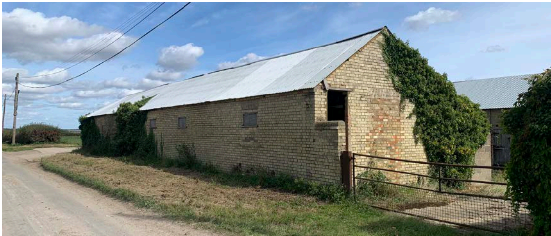
Figure 6. West elevation of west wing
