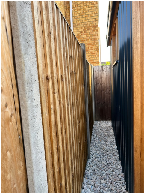
North elevation looking East.
