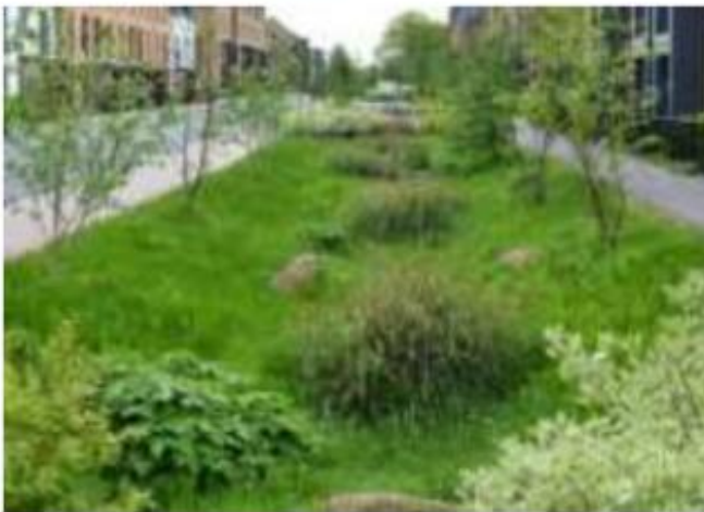
SuDS used to enhance streets
