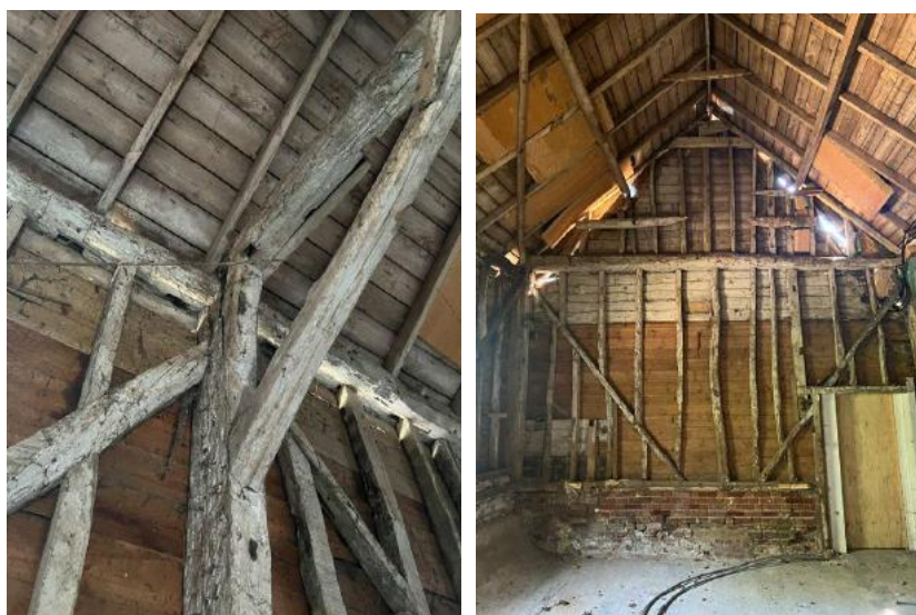
Figure 4. Photos of aspects of the original timber work, as seen from the interior
