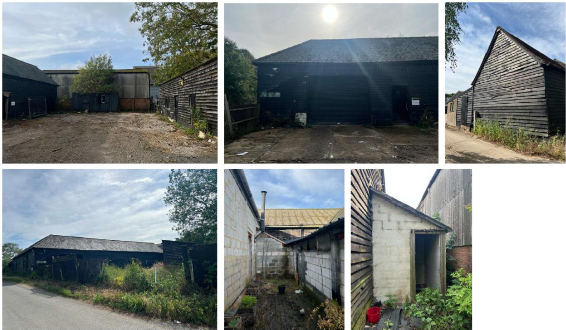
Figure 2. Photomontage of the exterior of the subject building
