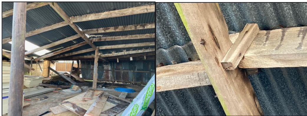
Photographs 13 - 14: Barn B - Corrugated iron roof
