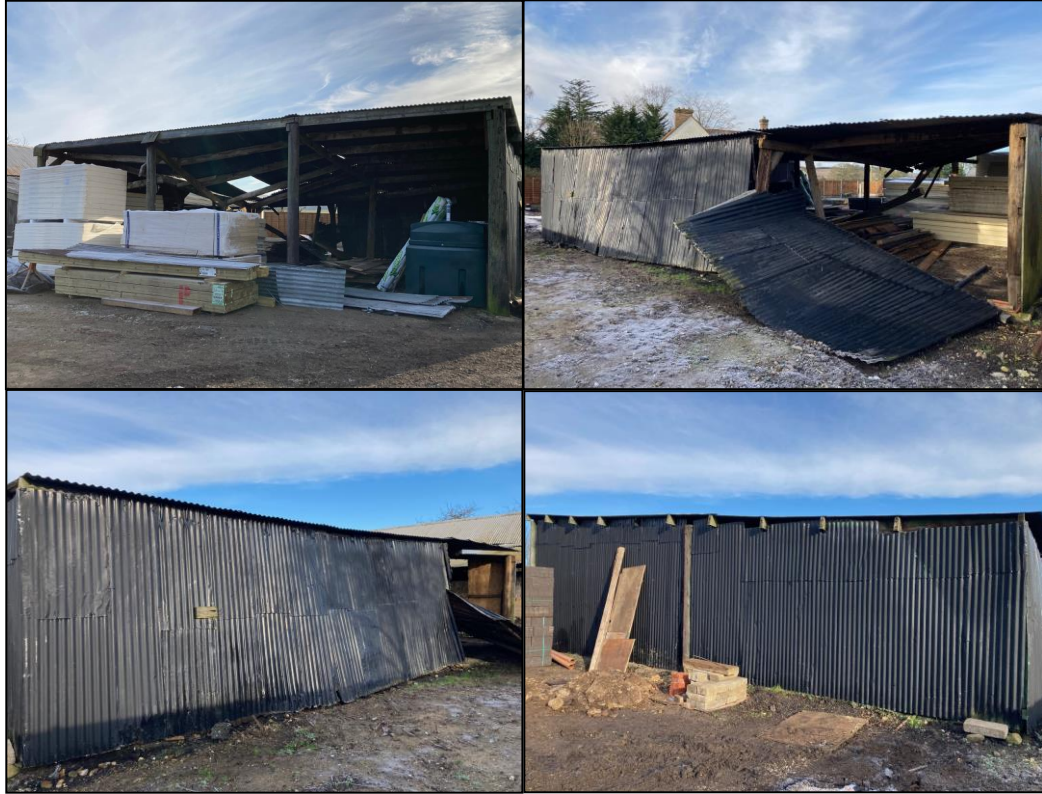
Photographs 9 - 12: Barn B - Front, rear & side elevations
