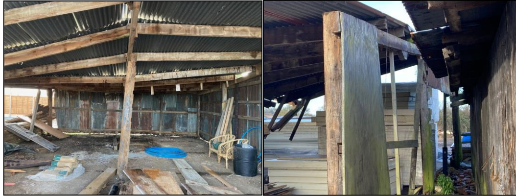
Photographs 15 - 16: Barn B - Internal void
