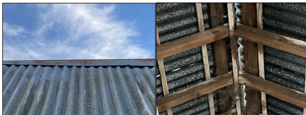
Photographs 5 - 6: Barn A - Corrugated iron roof
