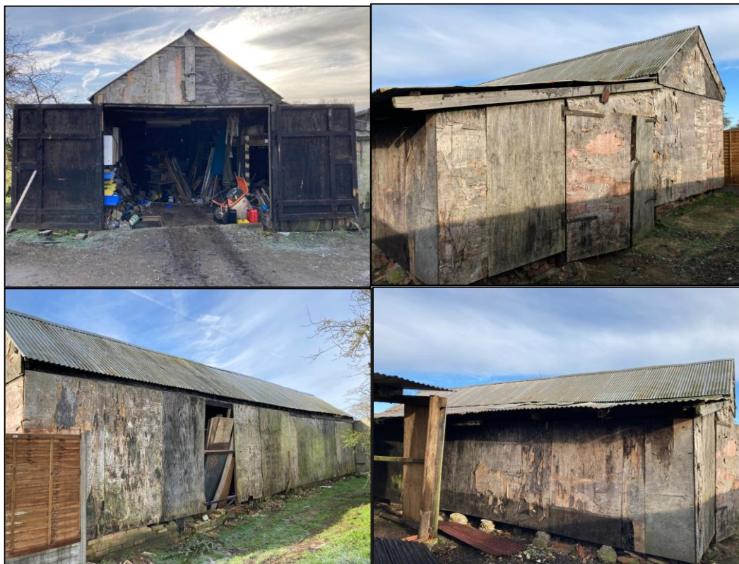
Photographs 1 - 4: Barn A - Front, rear & side elevations
