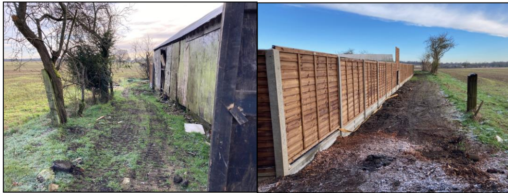
Photographs 21 - 22: Linear compartment to the rear of the new fence
