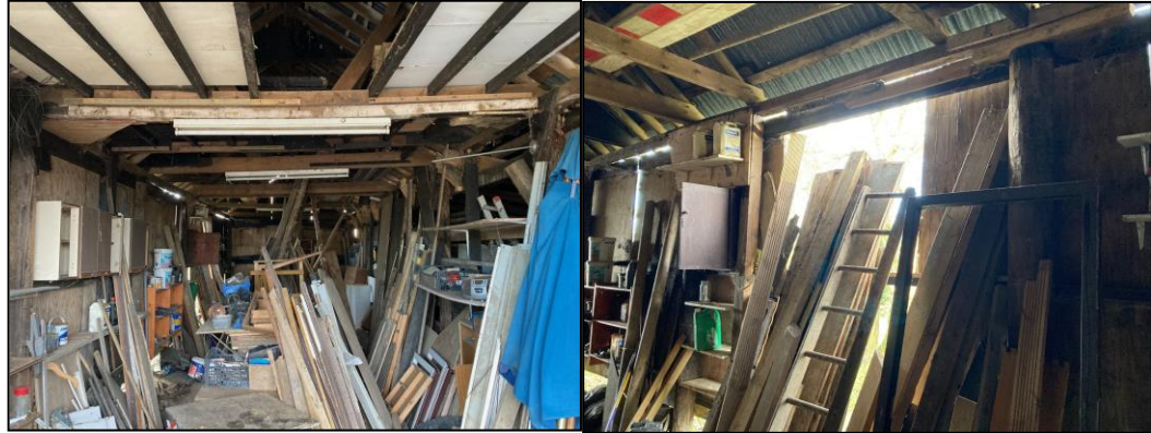
Photographs 7 - 8: Barn A - Internal void
