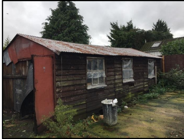
Photo 4.5: Building 1, exterior facing west.
