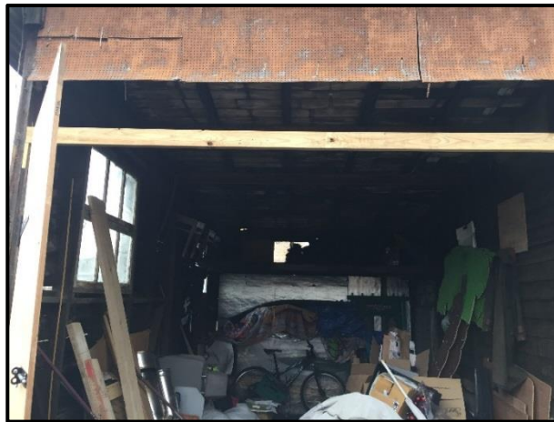
Photo 4.8: Building 2, internal storage area.
