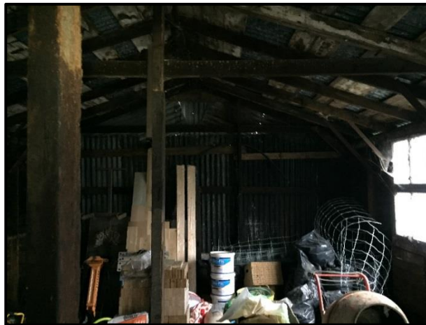
Photo 4.6: Building 1, interior facing north-west.
