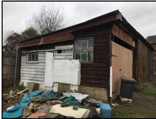
Photo 4.7: Building 2, western elevation.
