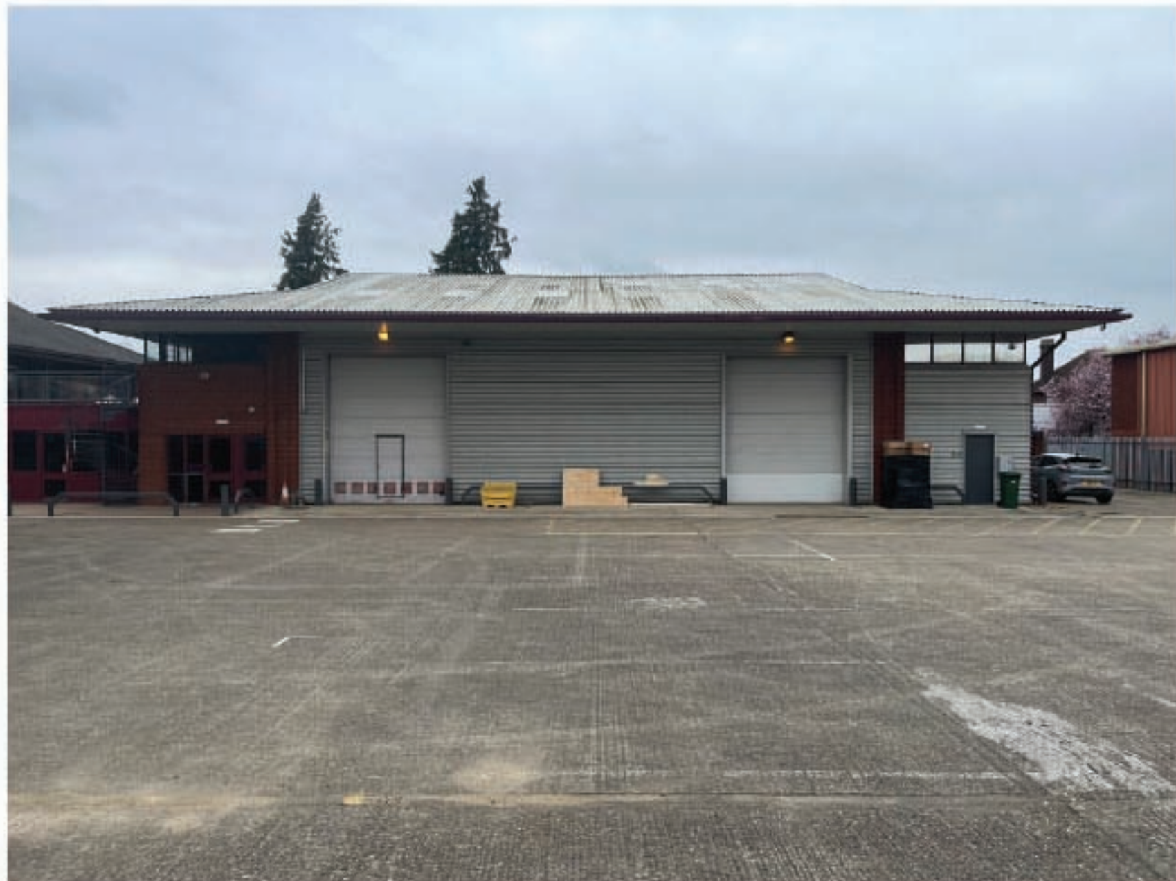
Photograph 4 Existing Factory Building
