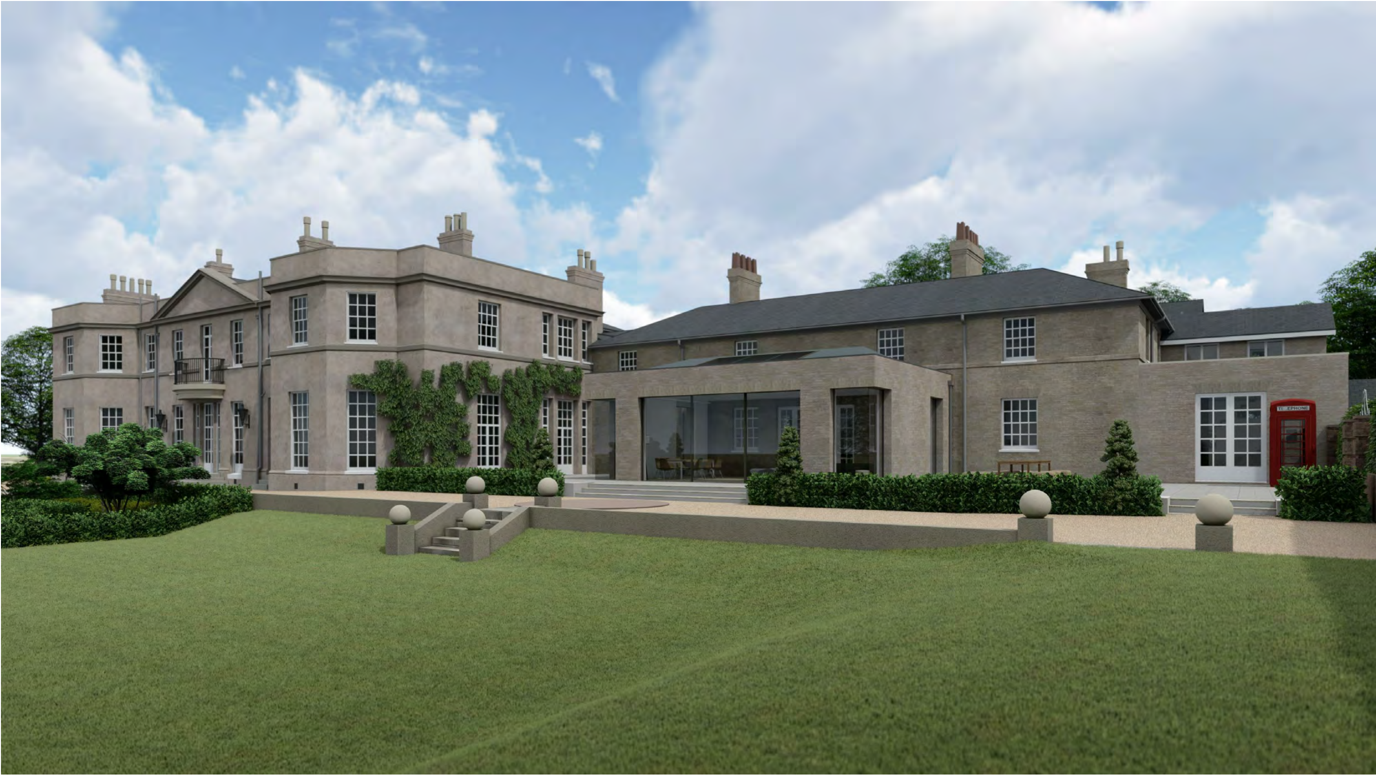
View of West Elevation
