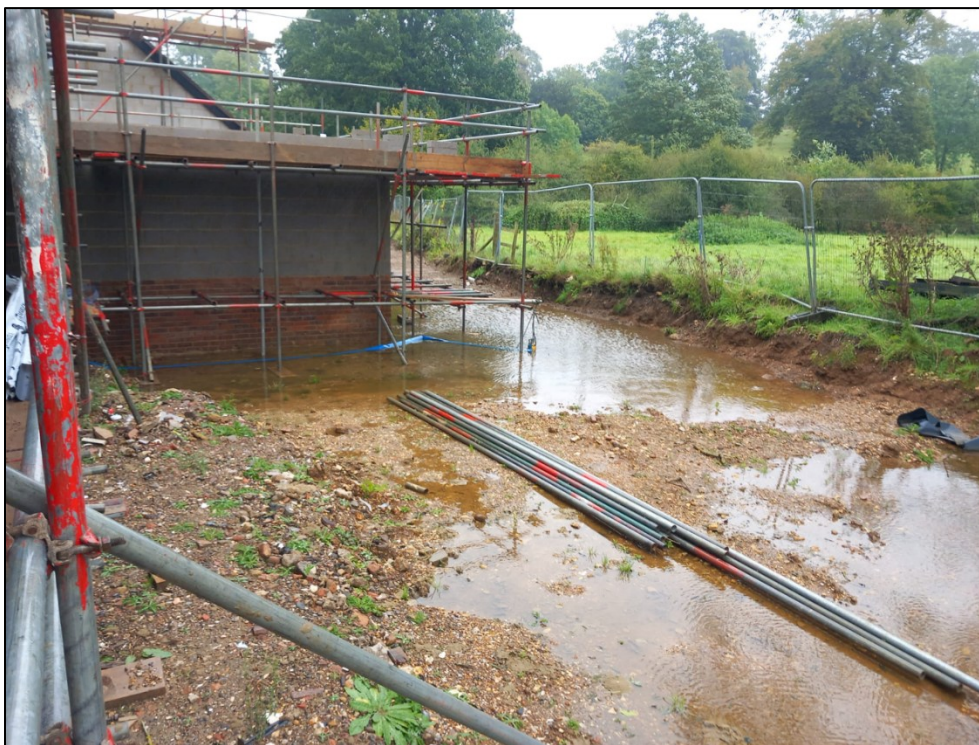
Plate 3: Southwest corner of site, facing northeast
