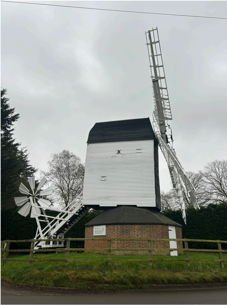
Plate 1. View looking south of Cromer Windmill
