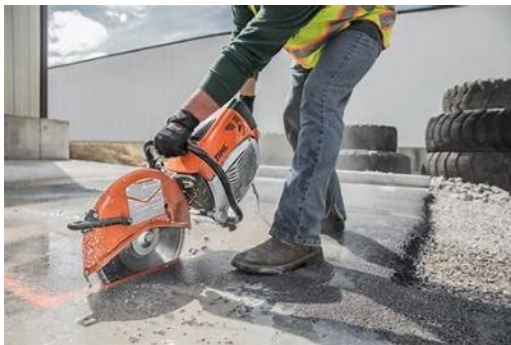
Figure 20 Saw with Dust Suppression
