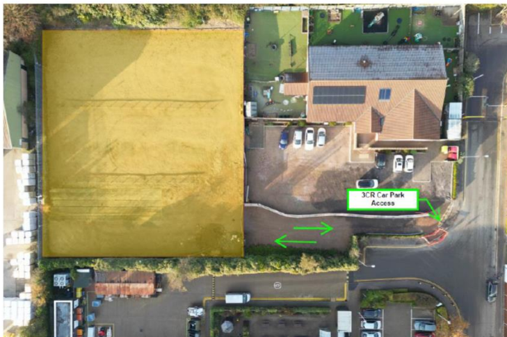
Figure 10 Sunhill Nursery Car Park
