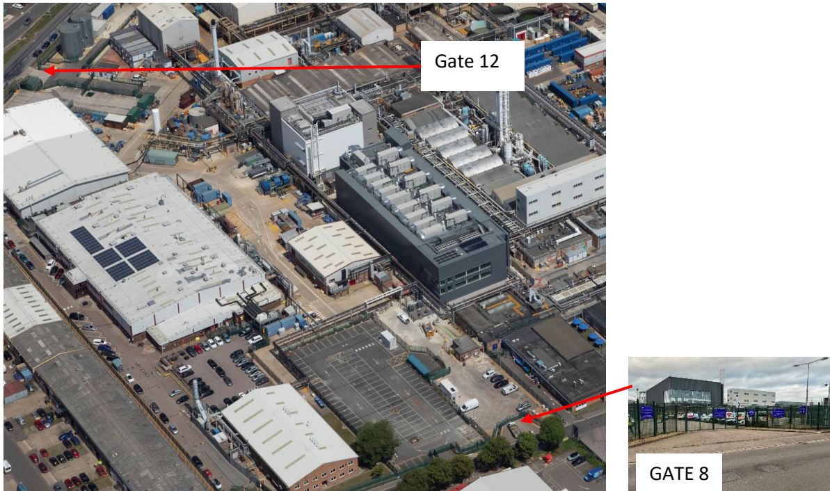
Figure 2 Gate 12 Adjacent to York Way
