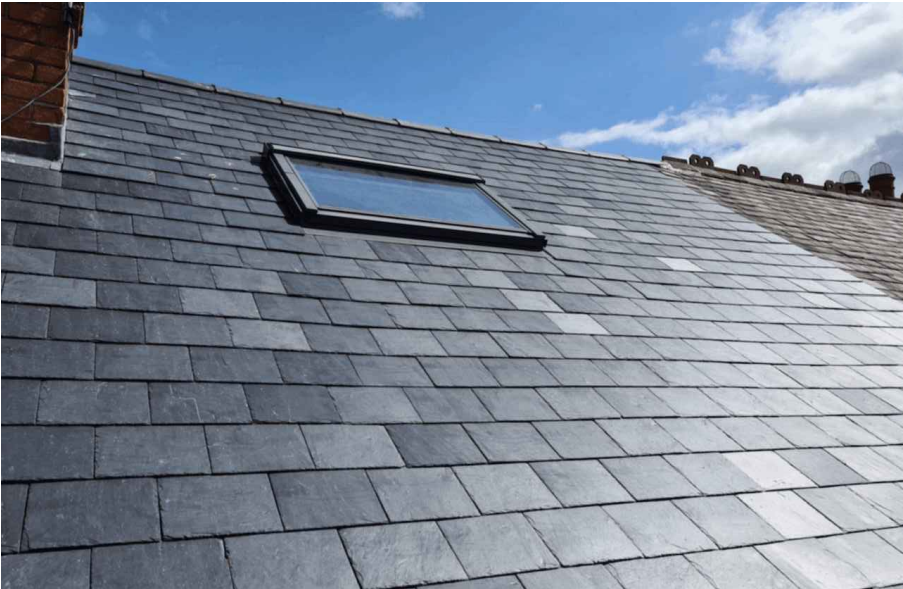
EXAMPLE OF SLATES TO MATCH EXISTING
