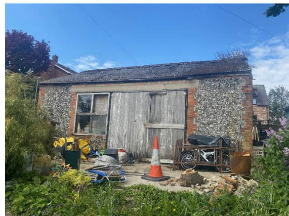
Photo of previous asbestos sheet roofing
