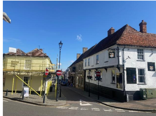
Photo of Front area and Buildings with clay plain tiles
