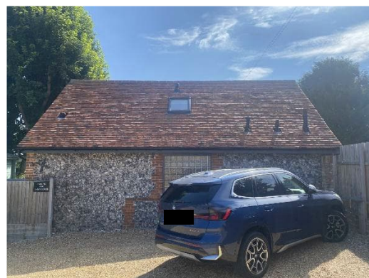
Barn Rear Photograph
