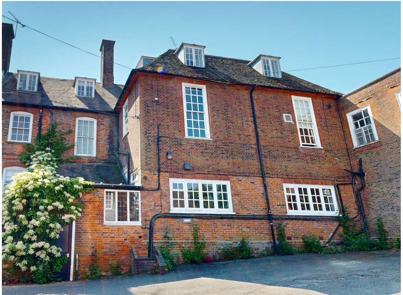
Present day photos of rear elevation East Annex and Stable Block
