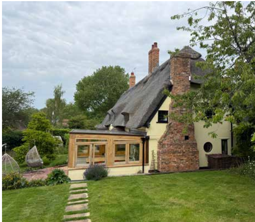
View from within the garden looking north towards the existing 2020 conservatory which adjoins the 1960/70s two storey extension to the south of Church Farm House
