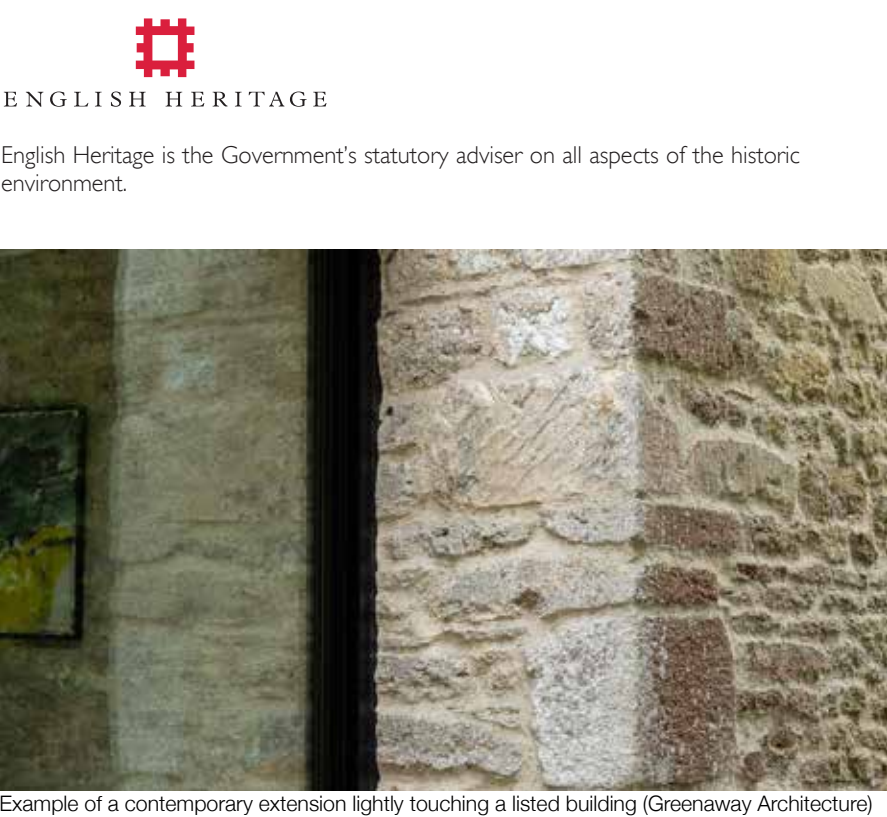
Example of a contemporary extension lightly touching a listed building (Greenaway Architecture)
