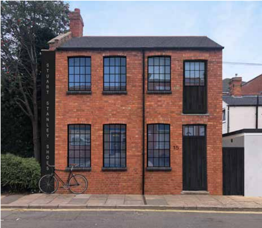
Greenaway Architecture - Conversion, refurbishment + extension of Listed Building Northampton
