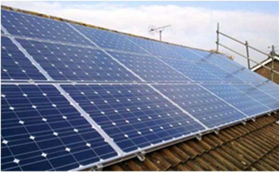
Figure 7.2 —Roof mounted PV panels
