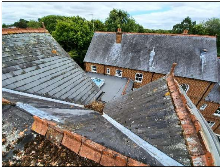
Photo 5: View over care home new wing (east) from roof of old wing (west).
