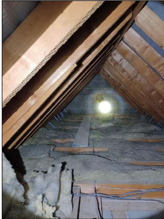
Photo 6: Interior of roof void.
