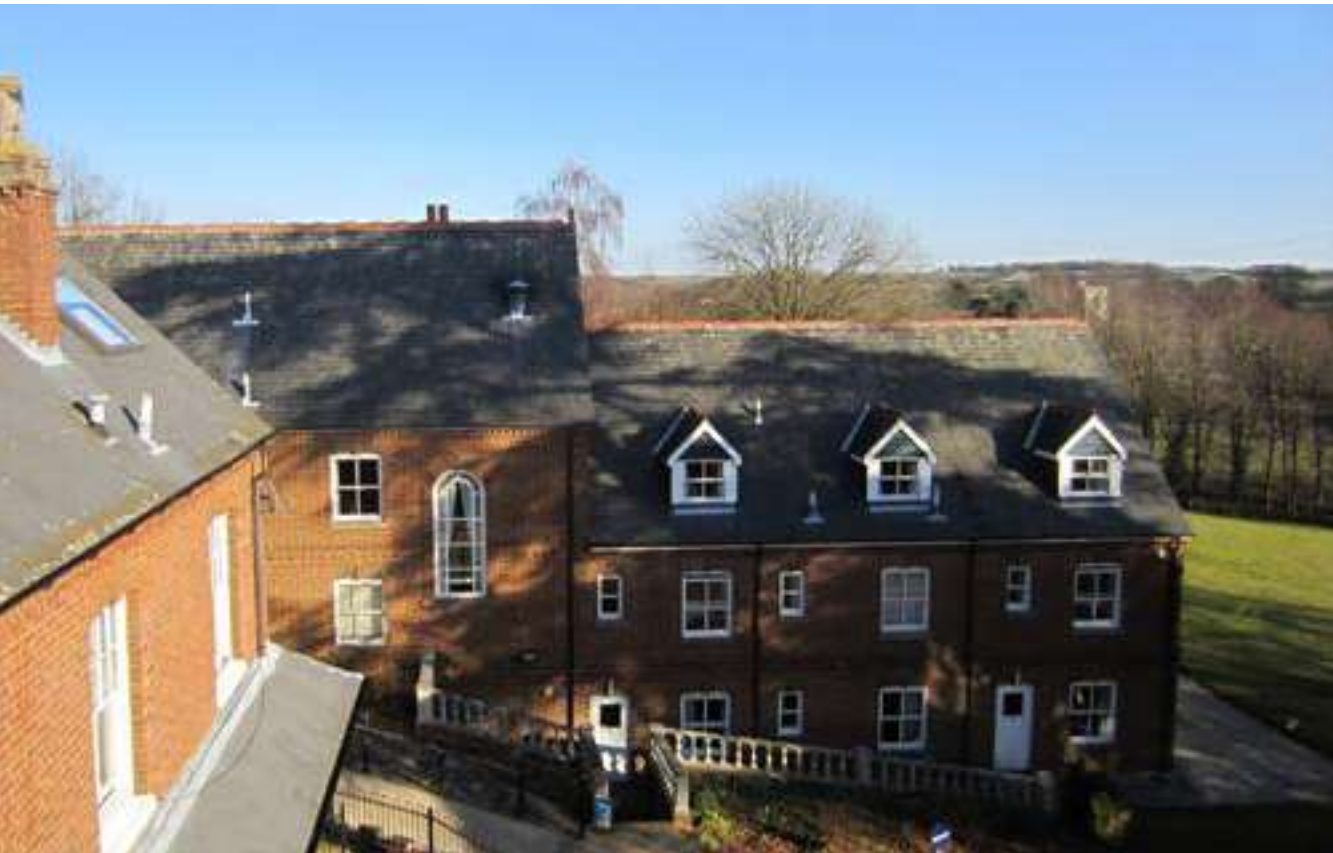
West Facade of 1990s Wing, Existing Guysfield Care Home
