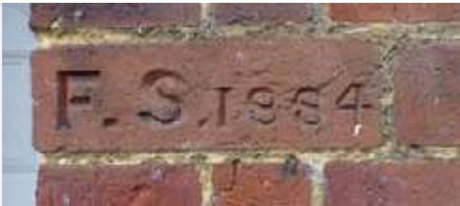
Inscribed brick to RHS of entrance porch
