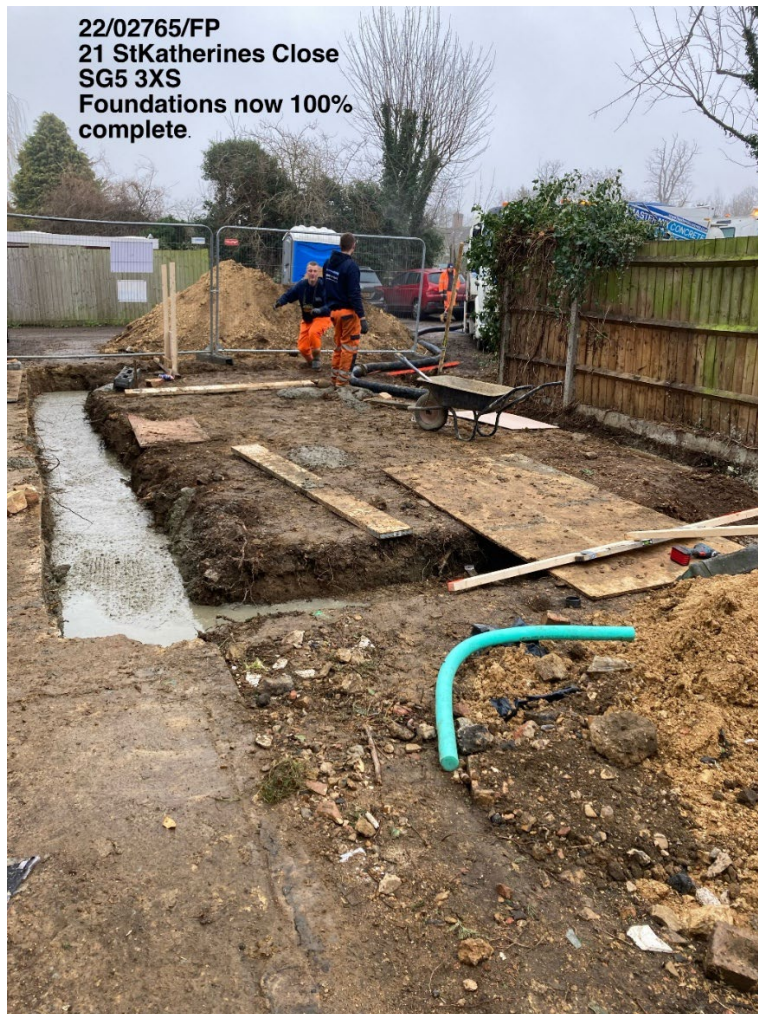
Foundations completed: Photo taken 09/01/2026
