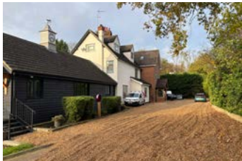
73 Park Lane, Main Building
