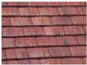
Marley Ashdown Handcrafted roof tile to match existing
