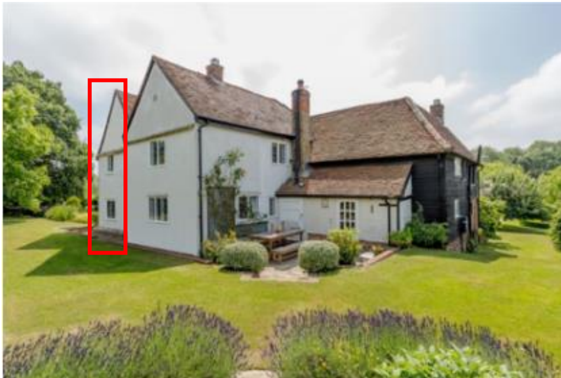
Figure 1 - Existing House showing elevation to be repaired
