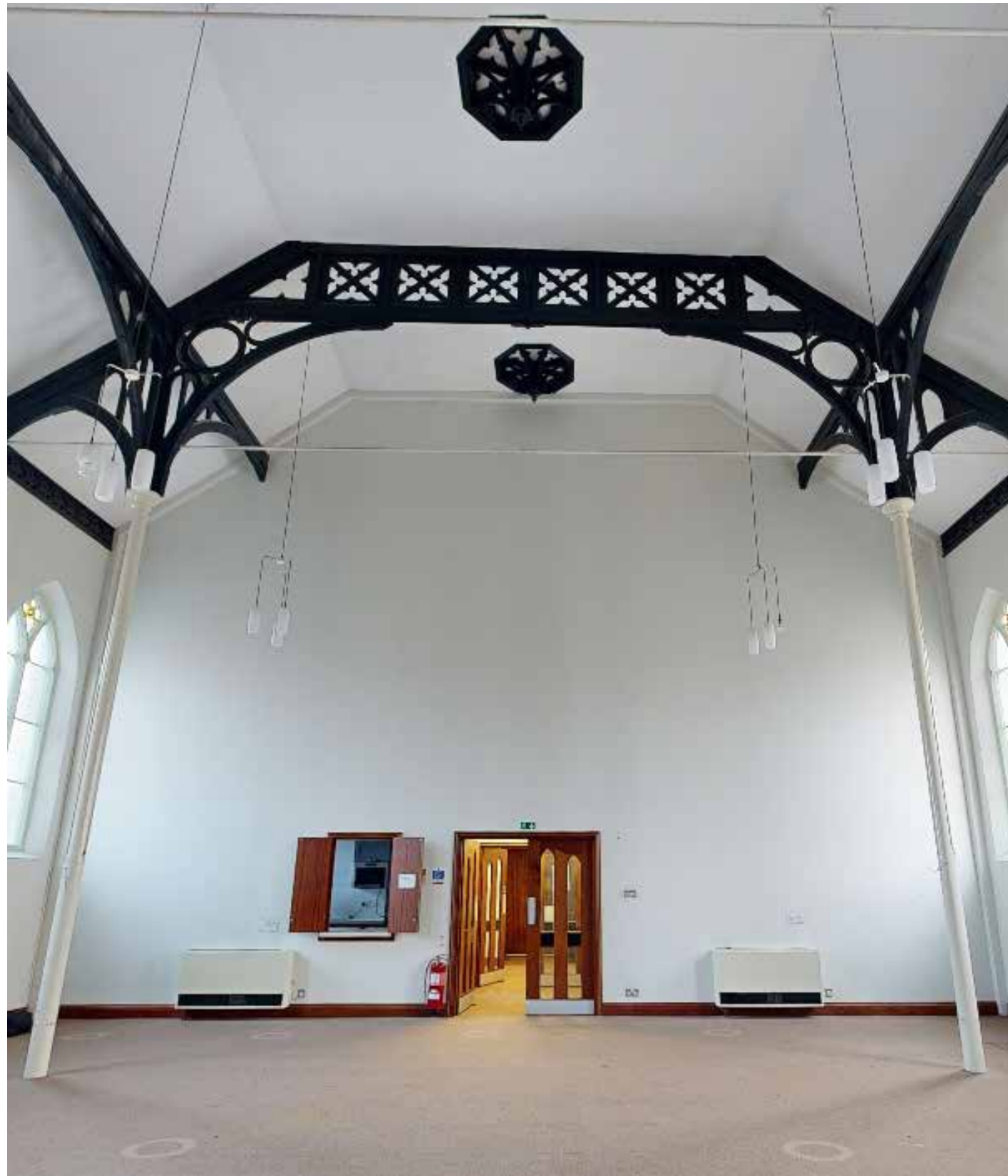
Fig. 10 : Internal view of the 1982-3 addition of the full height wall
