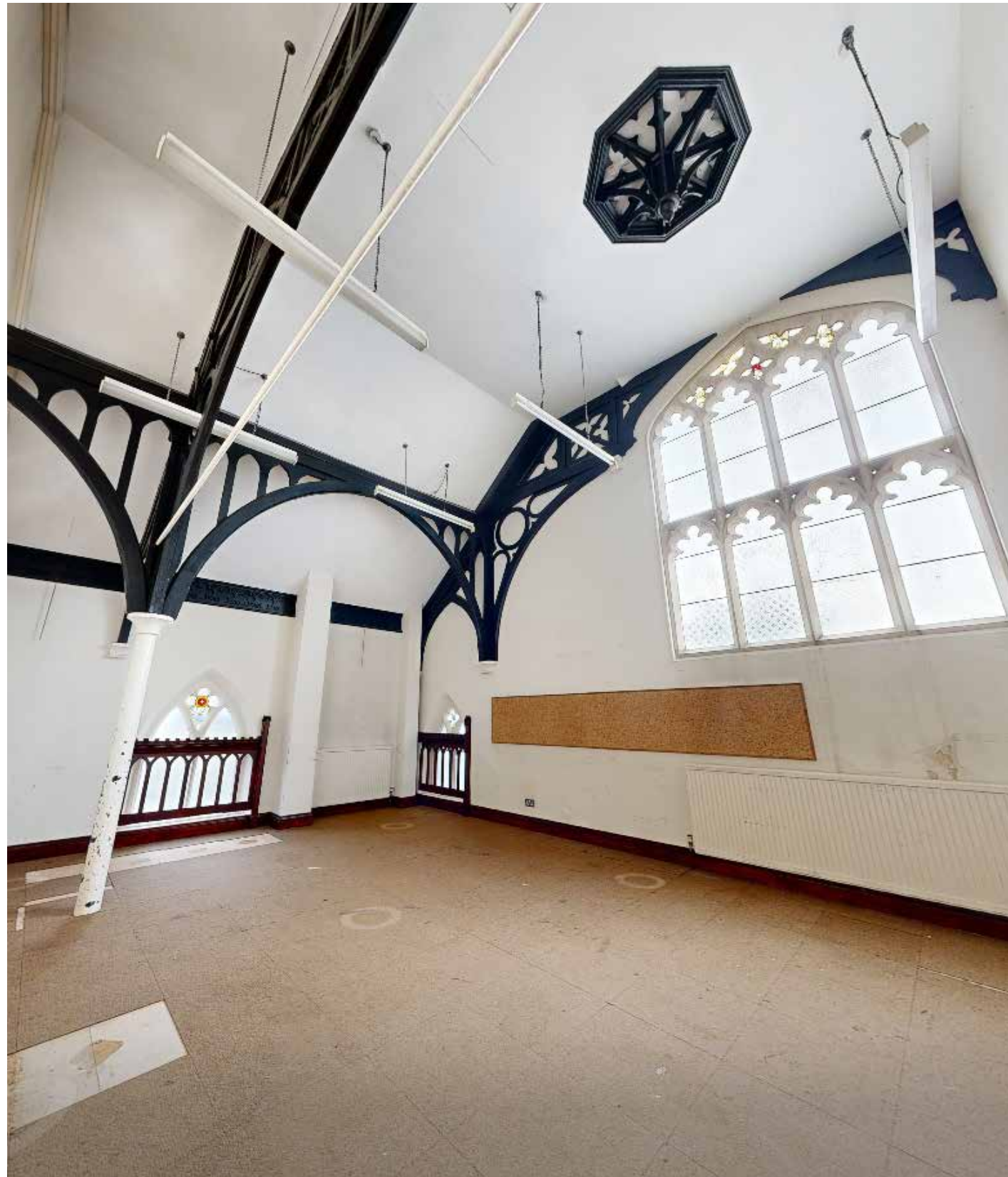
Fig. 15 : Existing photograph. Main feature window on the first floor
