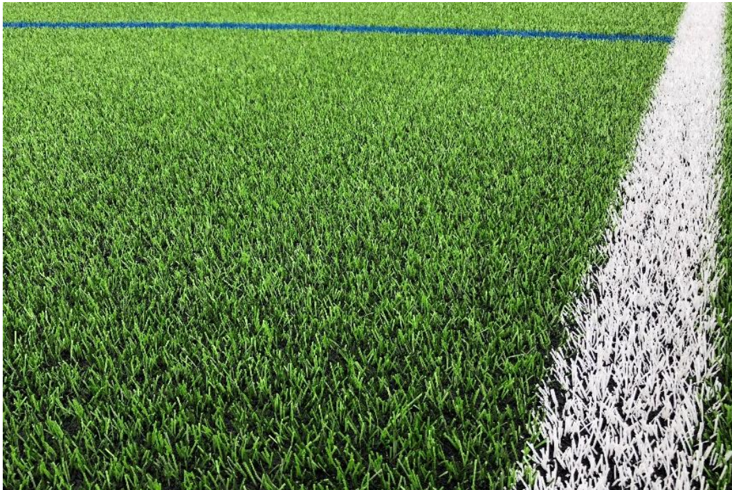
Figure 15 - Example 3G pitch with Rubber Crumb
