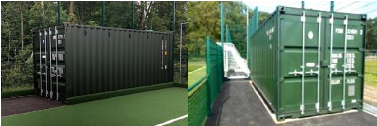
Figure 7 - A Typical Example of a Storage Container
