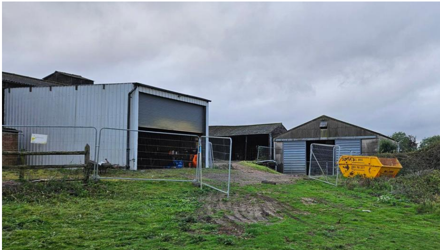
Modern steel barns to the west side of the complex
