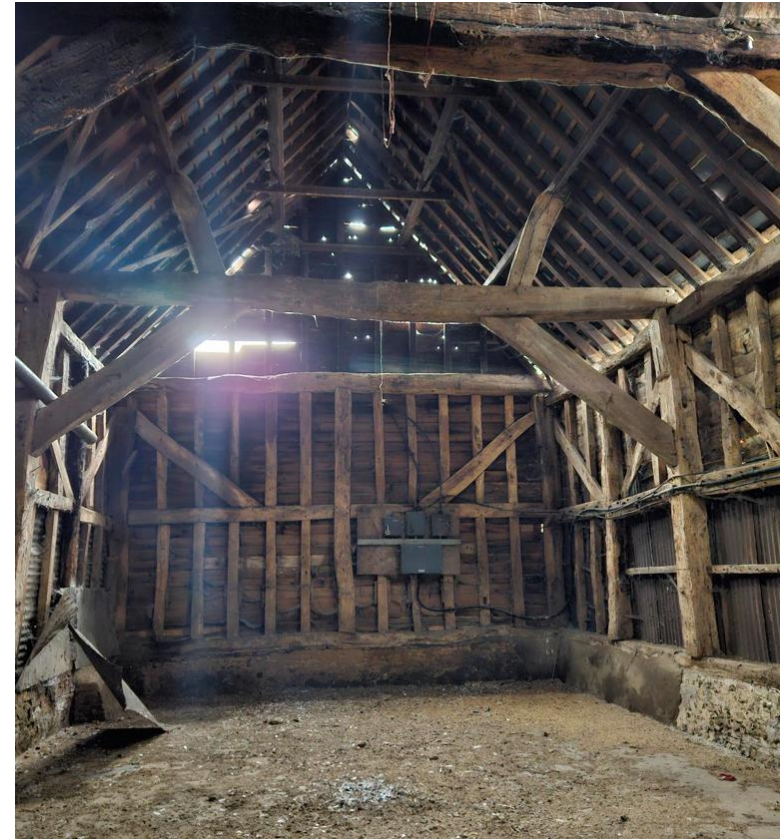
Internal view of the listed barn structure
