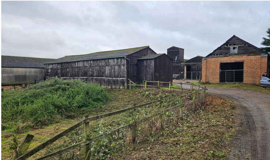
View on approach along the drive from the south
