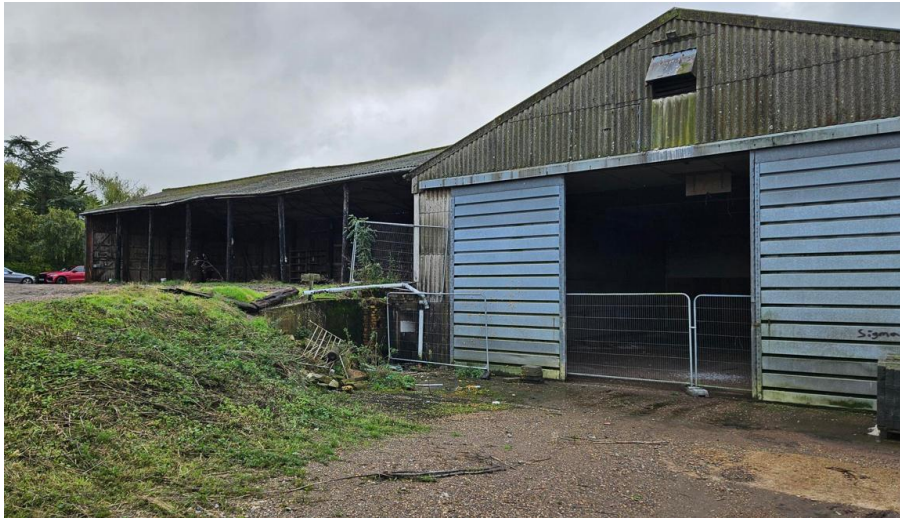
View showing the reducing levels from the cart shed to west side of site
