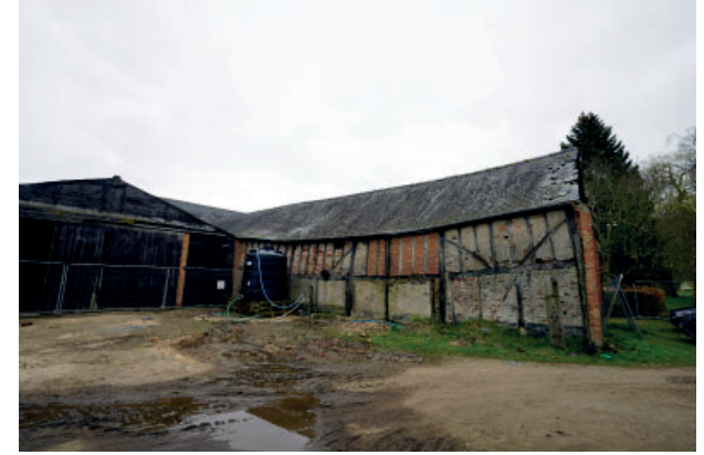
P3. View of barn 2 looking north east
