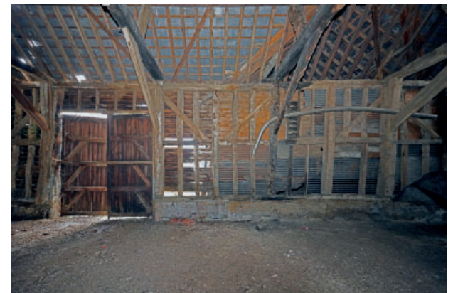
P12. Typical internal view of Listed barn (Barn 1)
