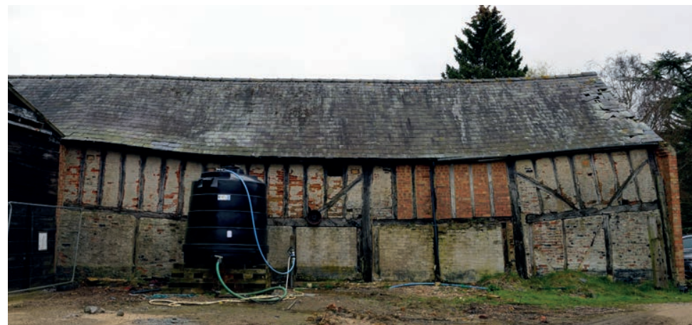
WEST ELEVATION OF BARN 2 SHOWING TIMBER FRAME WITH BRICK INFILL (IDENTIFIED AS ORIGINALLY OF 18th CENTURY CONSTRUCTION ON BORDER ARCHAEOLOGY PHASE PLAN)
