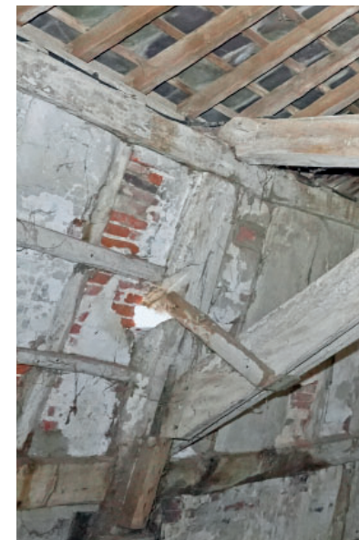
INCONSISTENT DETAILING OF WALL POSTS WITH BOTH JOWELED & PLAIN HEADS
