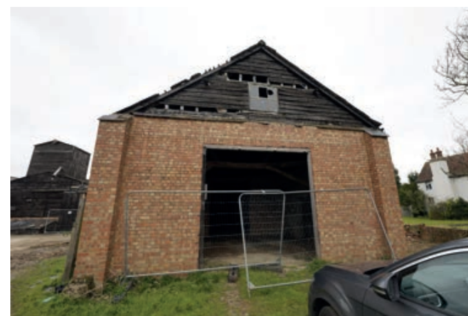
SOUTH GABLE RE-BUILT DURING 20th CENTURY
