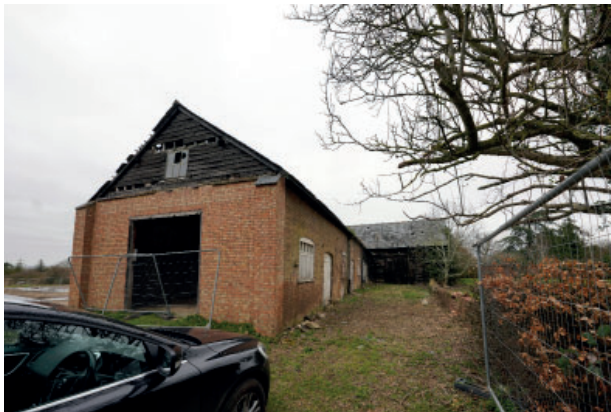
P4. View of barn 2 looking north
