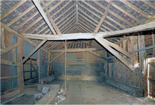
P13. Typical internal view of barn 2
