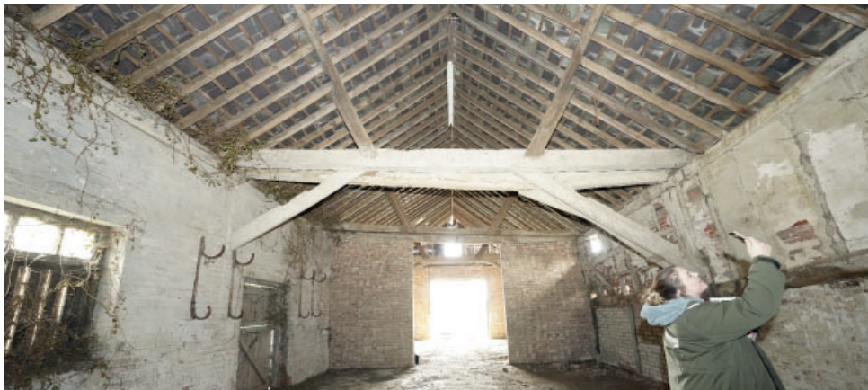
REPLACEMENT SOFTWOOD RAFTERS CARRIED ON OLDER ADAPTED TIE BEAMS AND RESIDUAL RETAINED ELEMENTS OF OLDER TIMBER FRAMED STRUCTURE.
