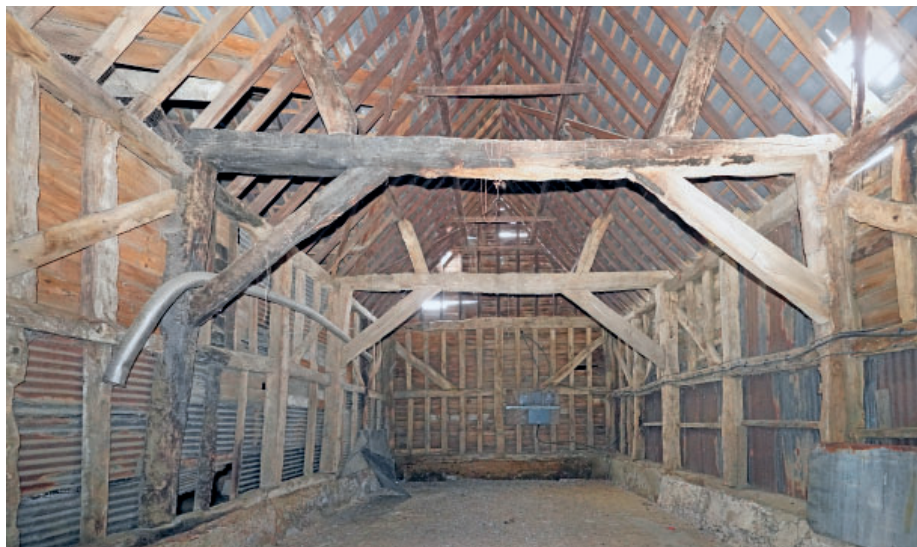
INTERIOR VIEW OF LISTED 17th CENTURY BARN SHOWING REPLACEMENT SOFTWOOD ROOF STRUCTURE ABOVE ORIGINAL BOX FRAME
