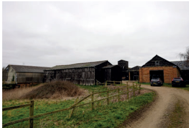
P5. View of barn group looking north west
