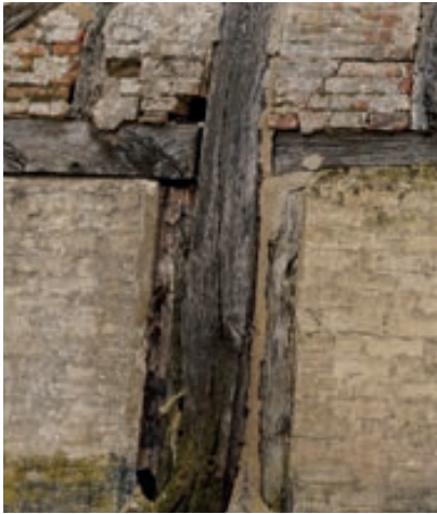
ADJOINING WALL POSTS. RIGHT HAND POST HAS PEG HOLES TO SECURE TENNONS OF MID-RAIL. LEFT HAND POST HAS NO PEG HOLES WITH POSSIBLE CRIPPLE STUDS TO SUPPORT MID RAIL
