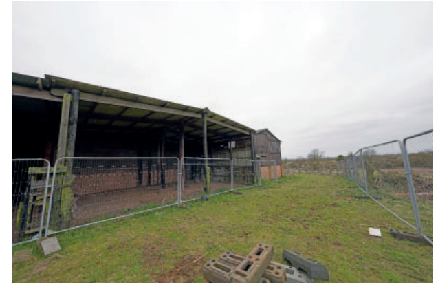
P9. View looking south west towards main barn group
