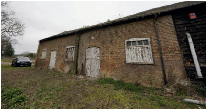
SOUTH END OF EAST ELEVATION IS OF LATE 19th CENTURY BRICK CONSTRUCTION
