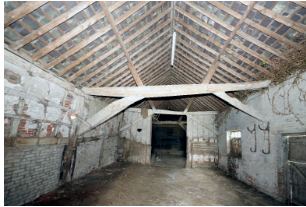
P14. Typical internal view of barn 2
