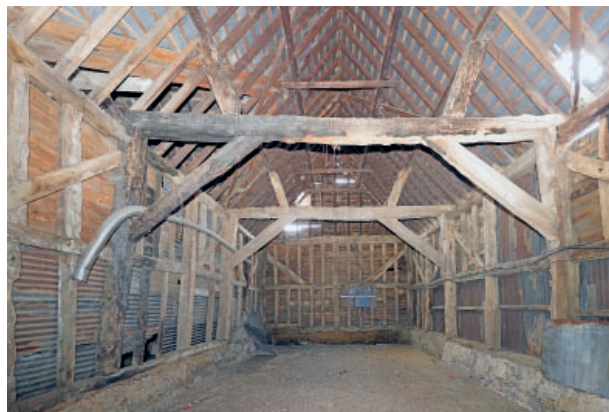
P11. Typical internal view of Listed barn (Barn 1)
