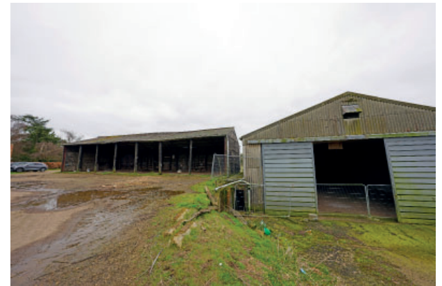
P6. View from within central yard looking south east
