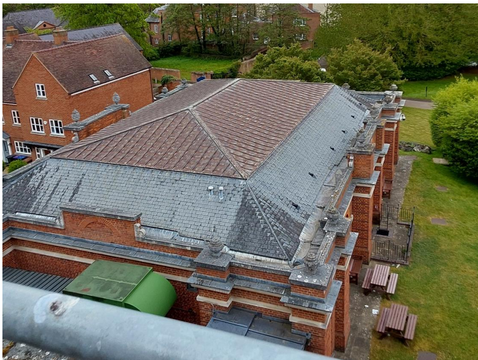
Photograph 6: North-eastern section of roof
