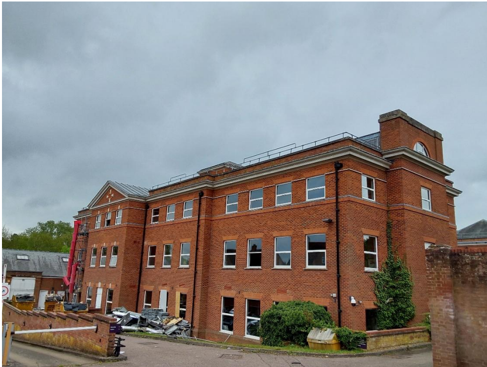
Photograph 3: Radcliffe House (north-west aspect)
