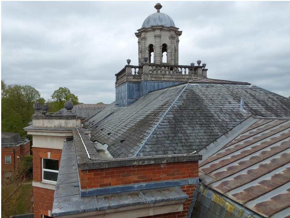
Photograph 5: Central section of roof
