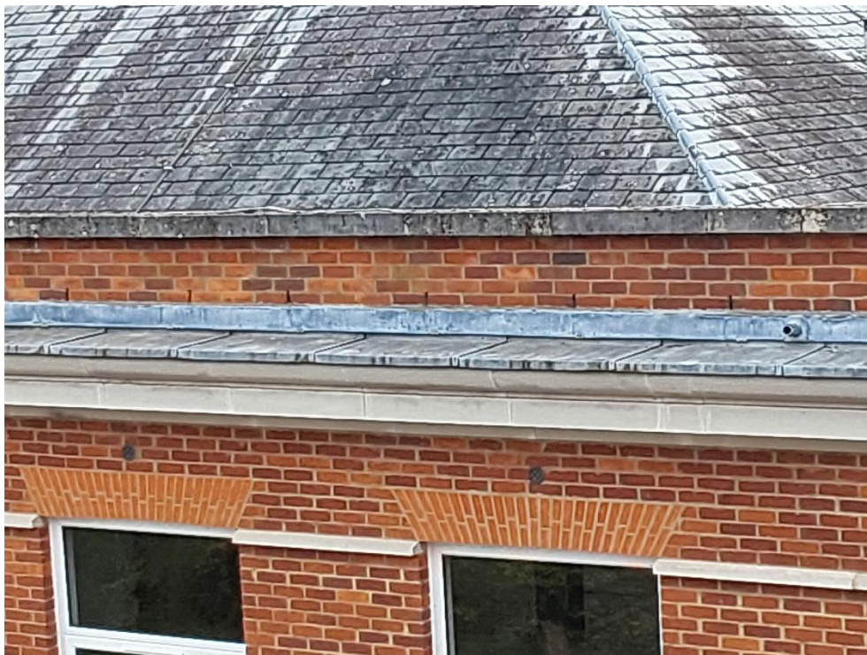
Photograph 7: TN1 – Weep vents in brickwork at the top of the wall
