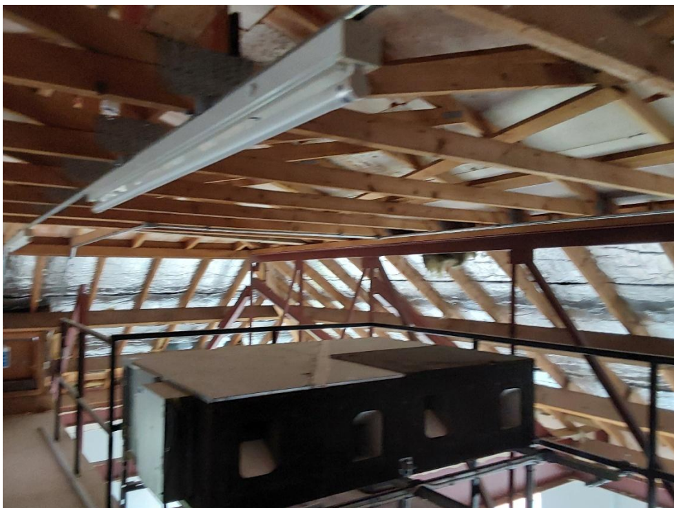
Photograph 14: Internal view of the main central roof cavity
