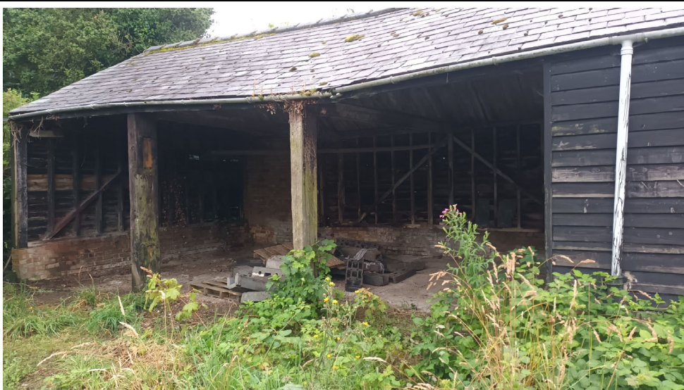
Photo 4: View to the southeast showing the northeastern corner of the barn
