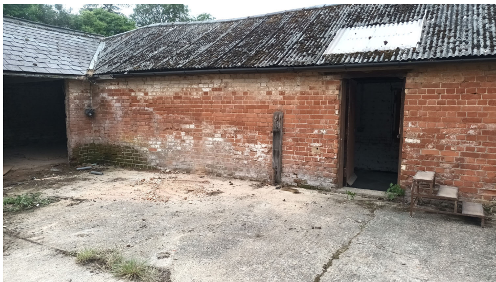
Photo 3: View to the southwest showing the location of CT02 within the courtyard
