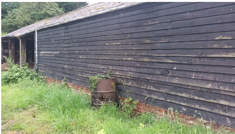
Photo 7: View to the southeast showing the northeastern corner of the barn
