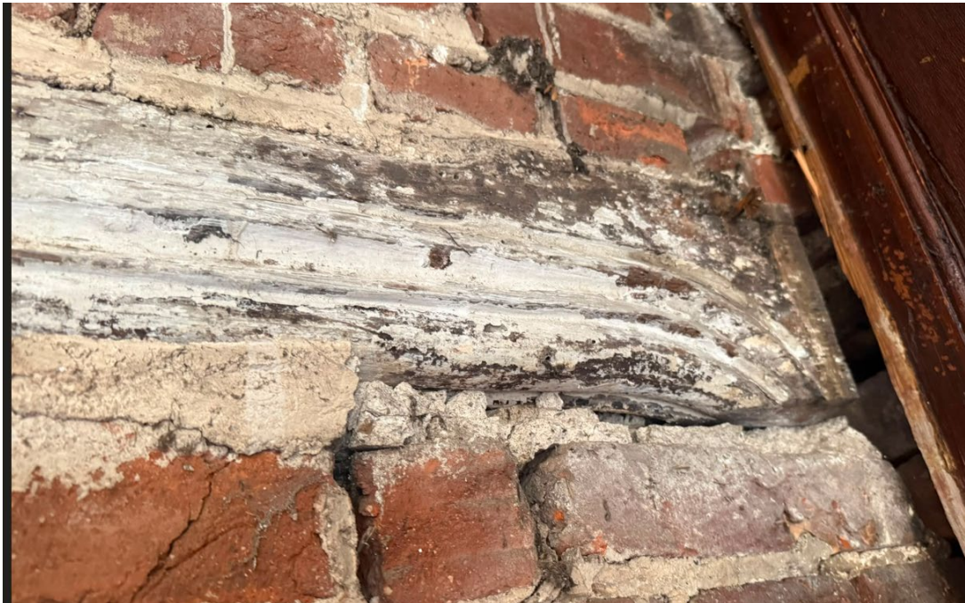
Detail of moulded embedded beam
