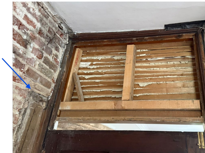
The modern doorway obstructs the decorated access to the stair tower. By not reinstating this doorway and leaving a larger opening within the dividing wall, the stair tower will be clearly legible.
