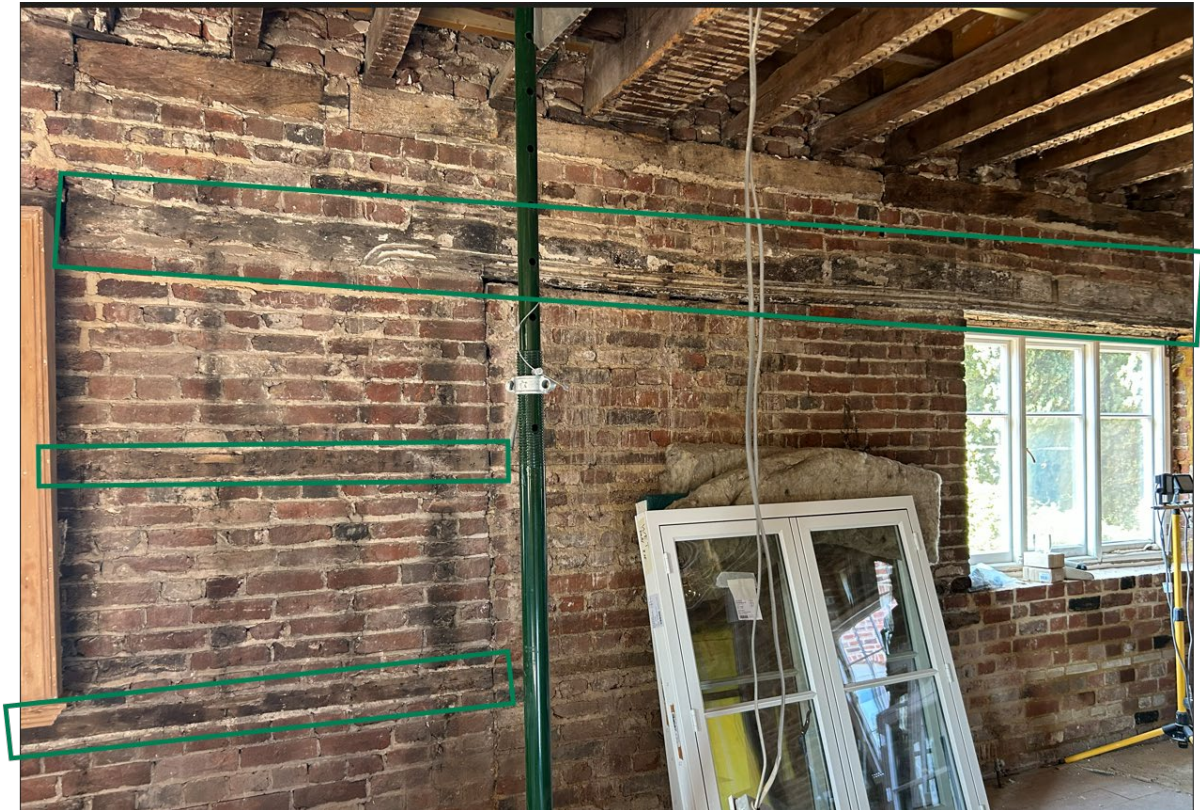
Detail of moulded embedded beam
