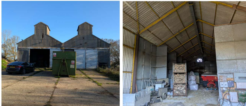
Figure 6 & 7 – Photographs of the Old Grain Store
